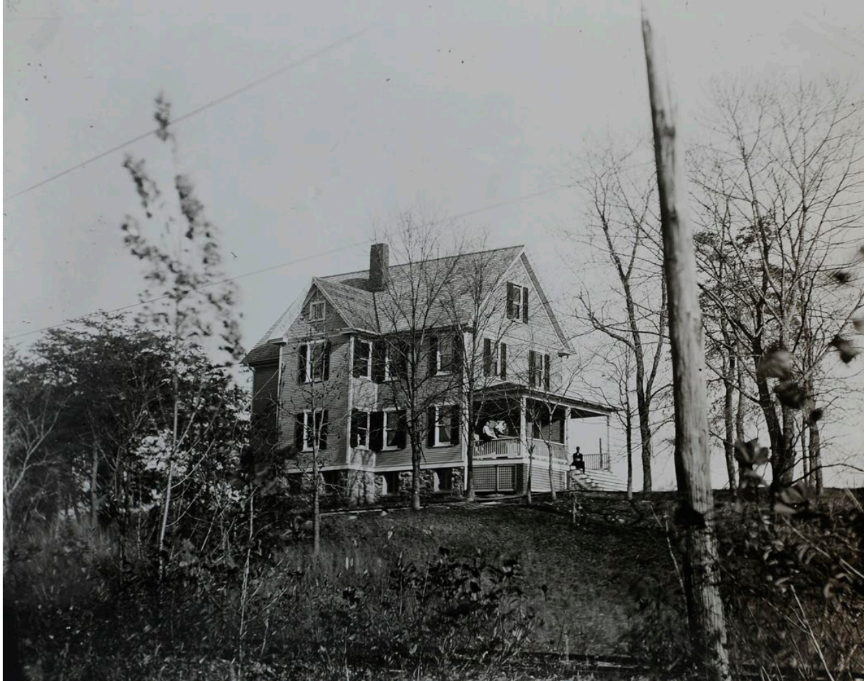
Figure 1: View of the Reynolds House, looking at the south (front) and west (side) elevations from the former Glen Echo Railroad line, ca. 1900.
