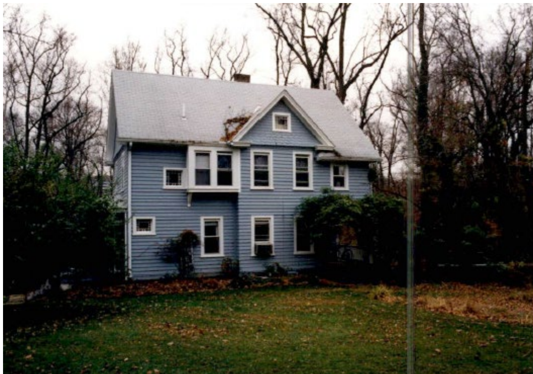
Figure 10: View of the Reynolds House, looking at the west (side) elevation, 1975. Source: Montgomery County Parks.
