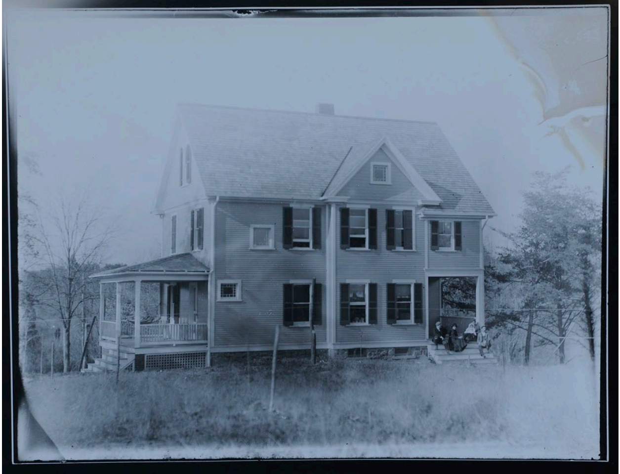
Figure 3: View of the Reynolds House, looking at the south (front) and east (side) elevations, undated. Source: Montgomery County Parks.
