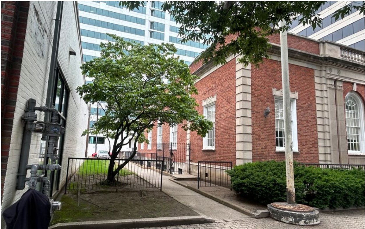
Figure 4: View of the south elevation of the historic building (May 2026, Historic Preservation Division).
