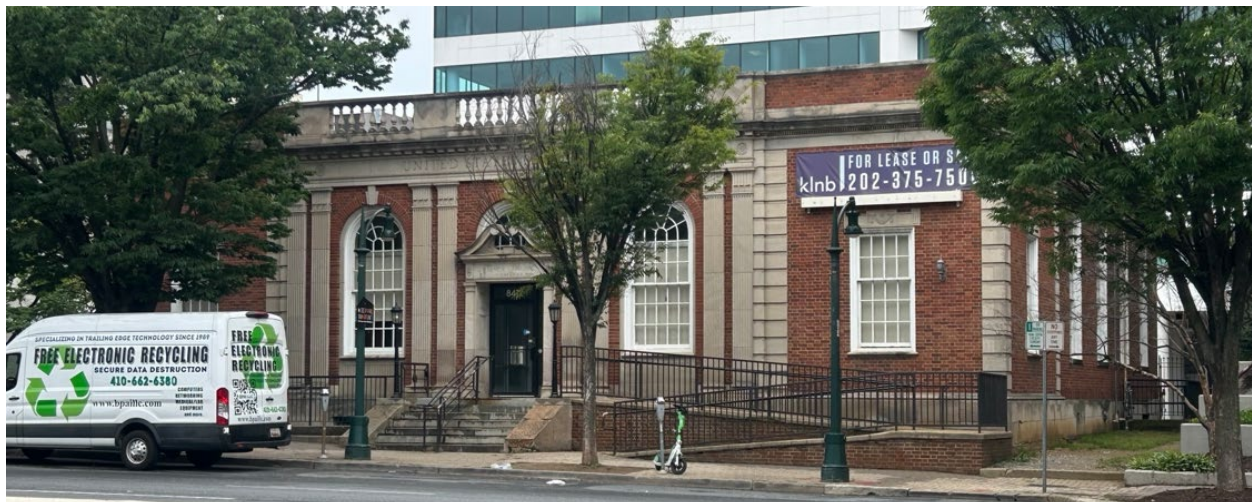
Figure 2: Front and partial north side elevations of 8412 Georgia Avenue (May 2026, Historic Preservation Division).
