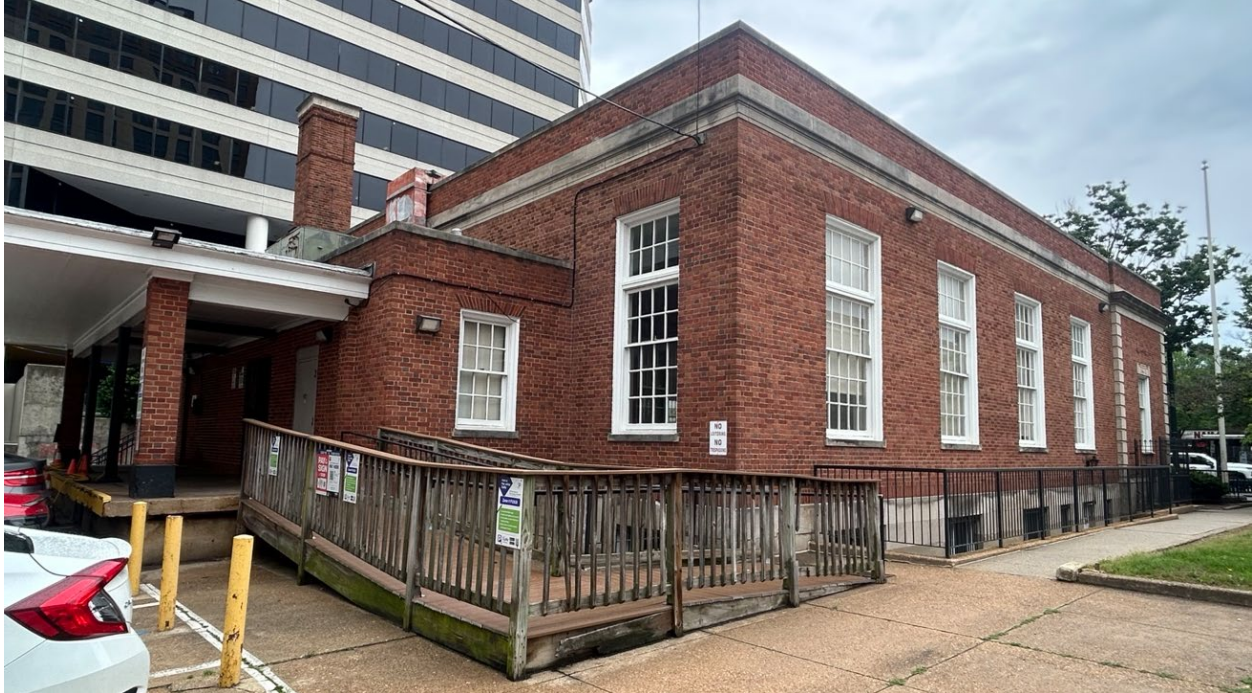
Figure 8: View of the south and rear (west) elevations of the subject property (May 2026, Historic Preservation Division).
