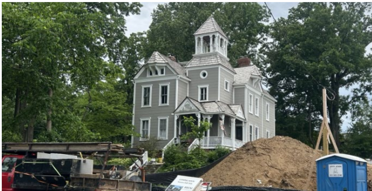
Figure 2: View of the front and west side elevations of the subject property from Holman Avenue.
