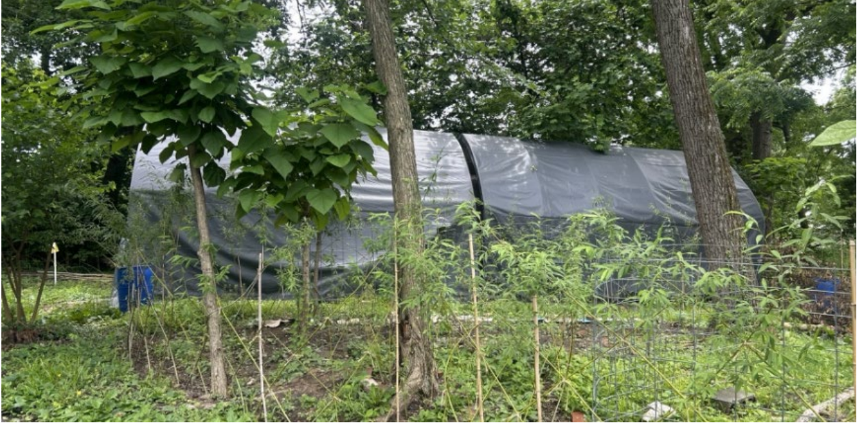
Figure 8: North side elevation of the structure(s) from Hollow Glen Place (May 2026, Historic Preservation Division).
