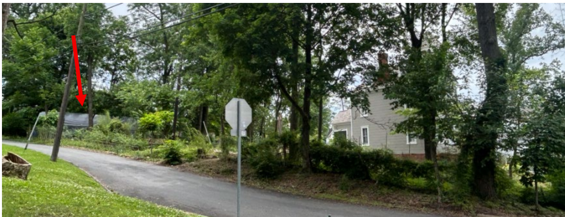
Figure 4: View of the subject property and the accessory structure from the intersection of Holman Avenue and Hollow Glen Place (May 2026, Historic Preservation Division).
