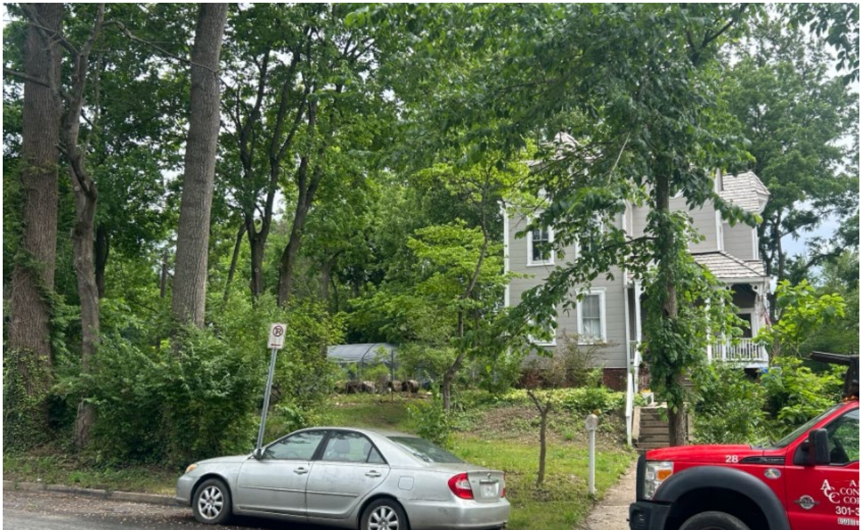
Figure 7: View towards the accessory structure(s) from Holman Avenue (May 2026, Historic Preservation Division).
