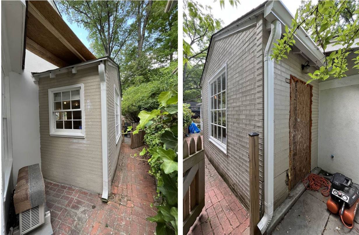
Figure 3: Addition with faux brick cladding.
