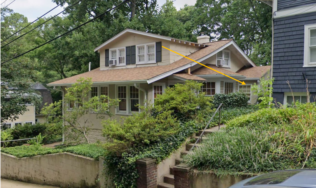
Figure 7: View of the subject property from the right-of-way along Valley View Avenue. The side addition is noted with a yellow arrow.
