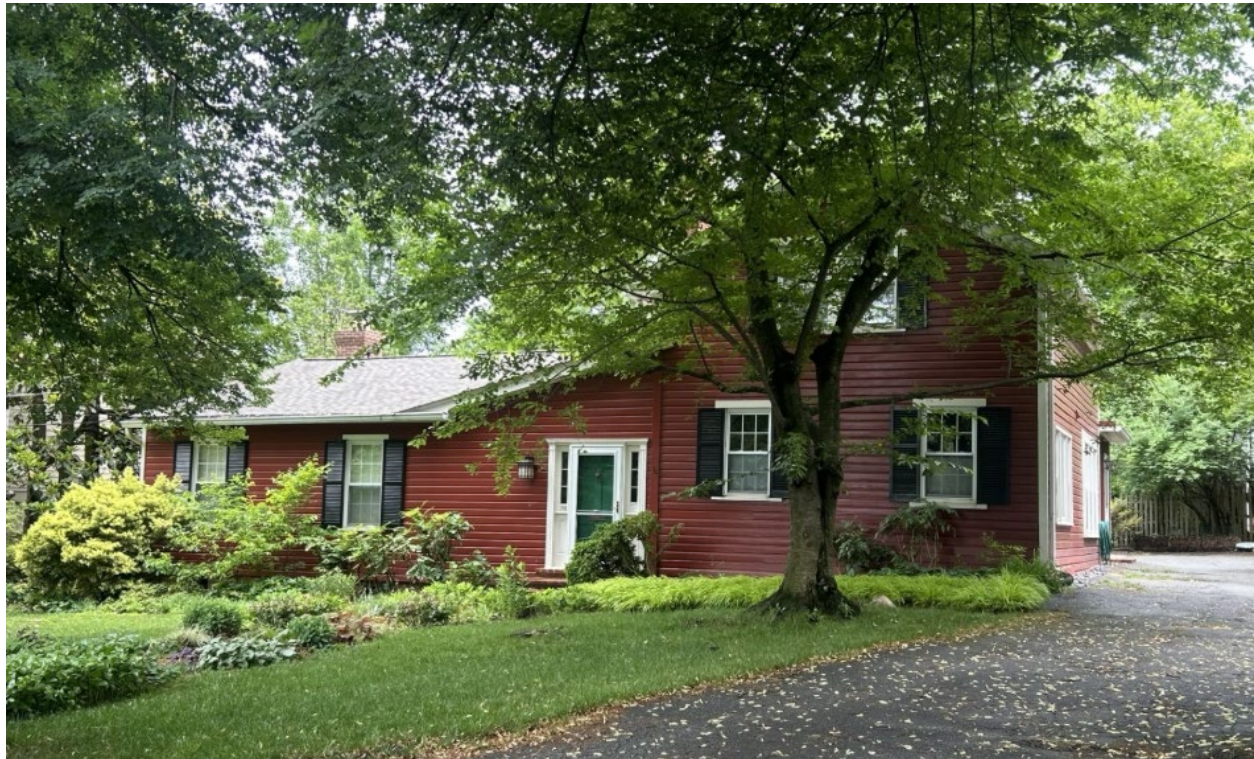
Figure 2: Front elevation of the subject property (May 2026, Historic Preservation Division).
