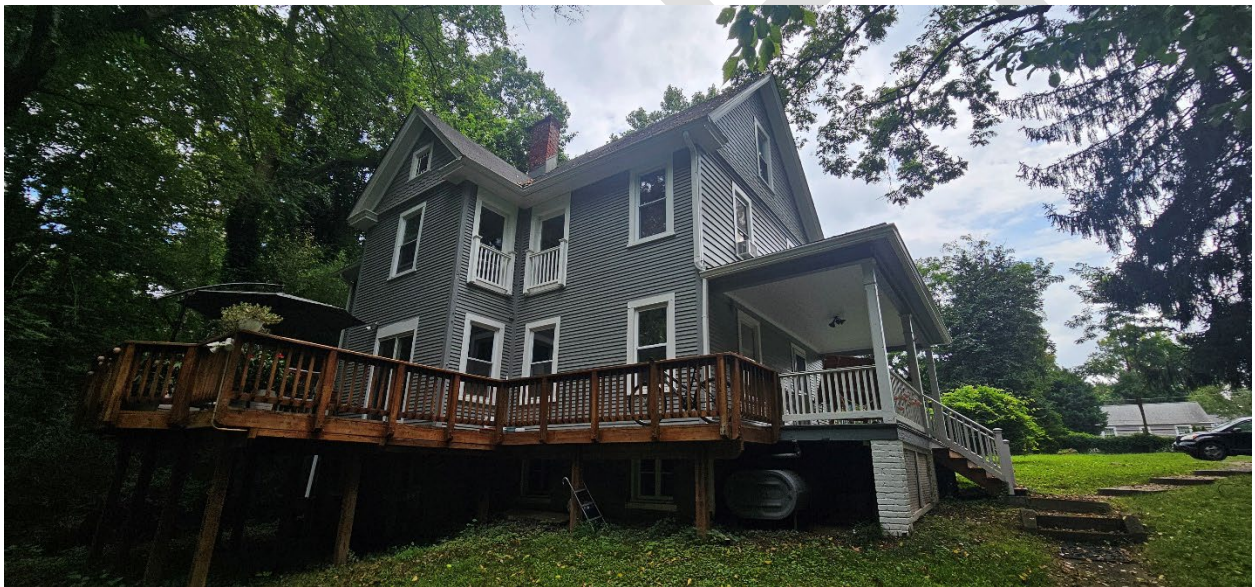
Figure 4: View of the Reynolds House, looking at the south (front) and west (side) elevations, 2025. Source: Montgomery Planning.
