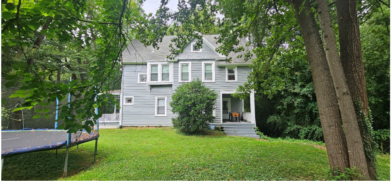
Figure 3: View of the Reynolds House, looking at the east (side) elevation, 2025. Source: Montgomery Planning.
