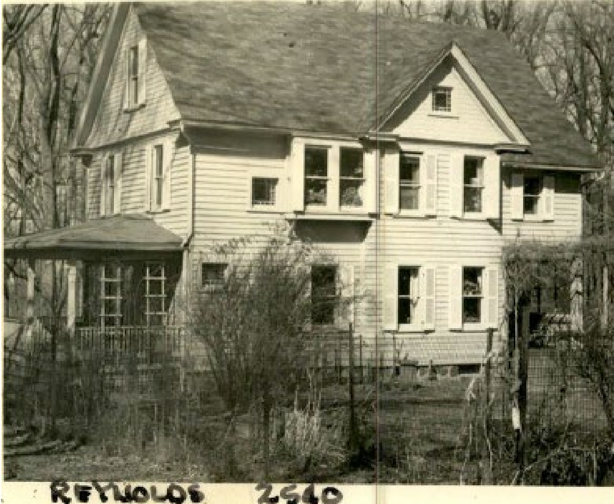
Figure 4: View of the Reynolds House, looking at the south (front) and east (side) elevations, 1970. Source: Montgomery County Parks.
