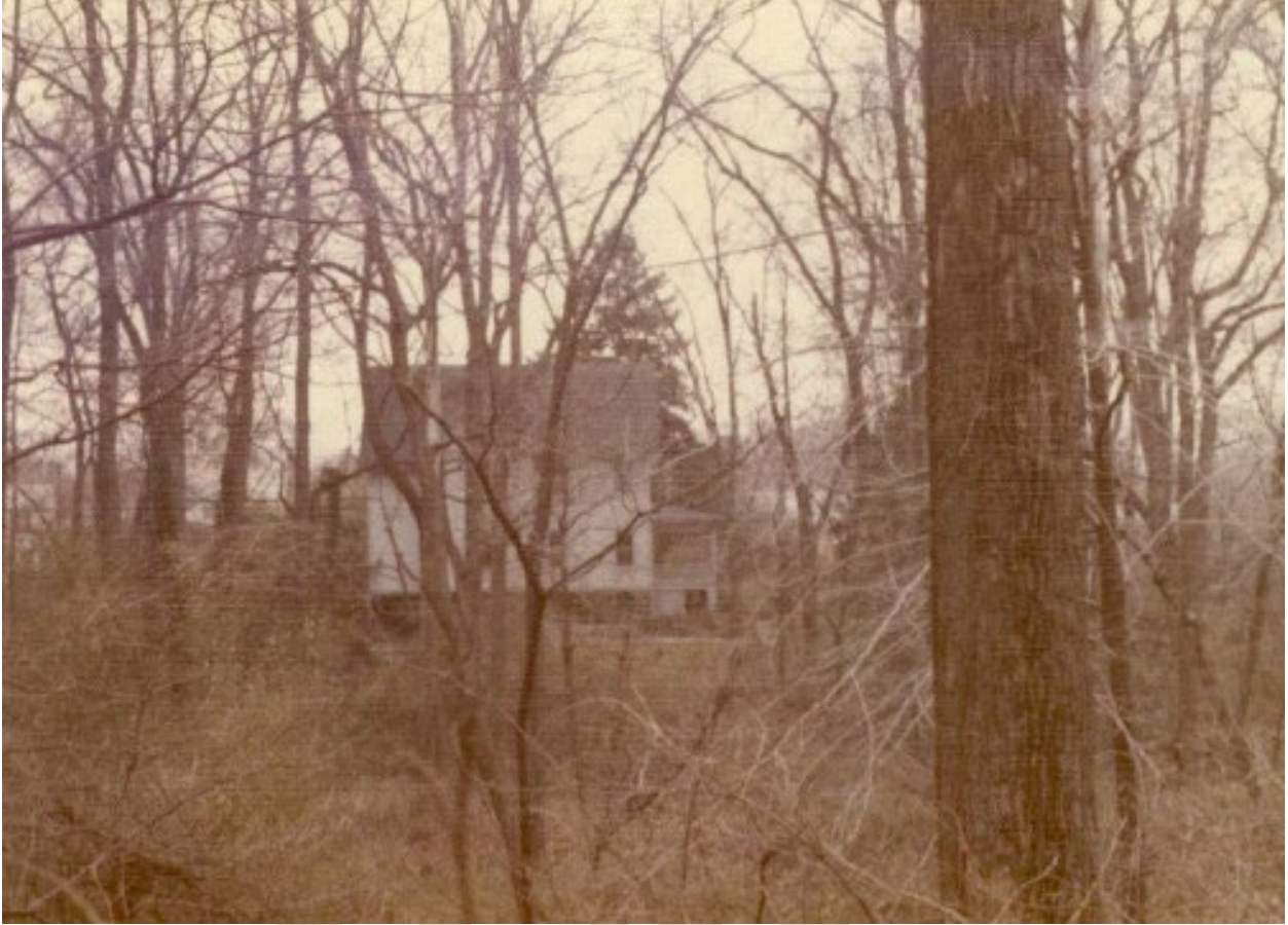
Figure 8: View of the Reynolds House, looking at the west (side) elevation from across Little Falls Branch, 1975. Source: Montgomery County Parks.
