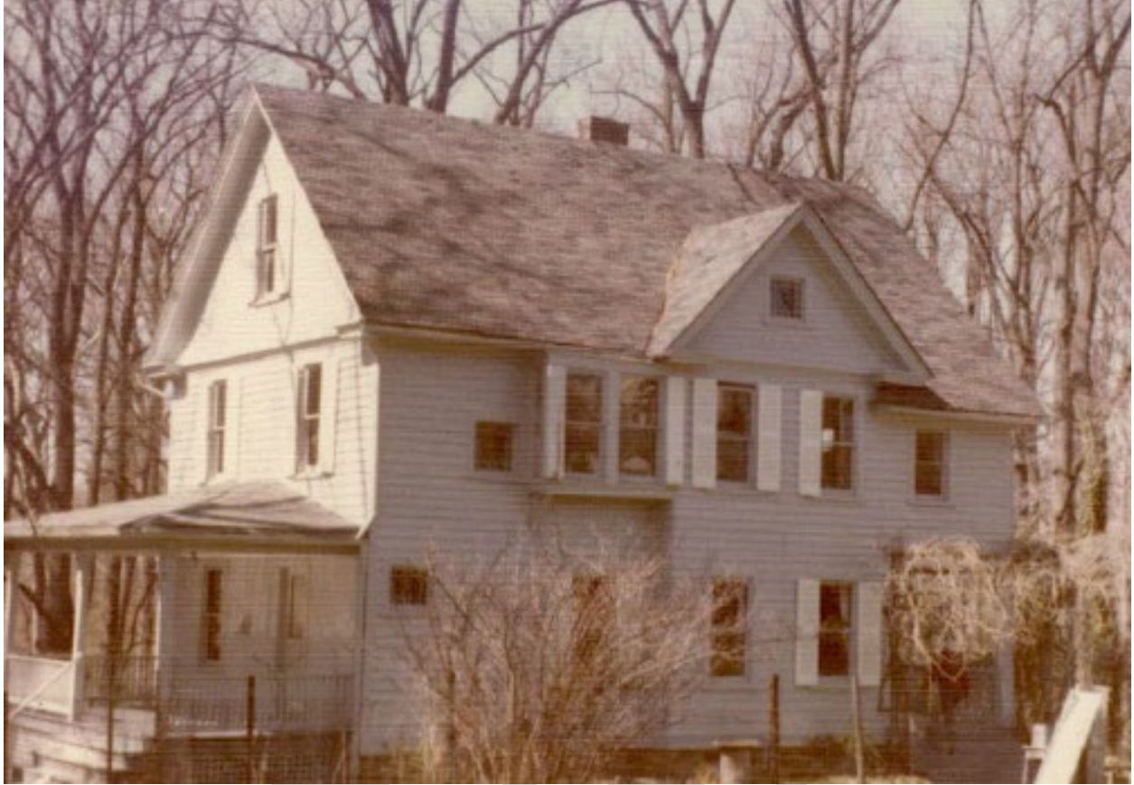
Figure 6: View of the Reynolds House, looking at the south (front) and east (side) elevations, 1976. Source: Montgomery County Parks.
