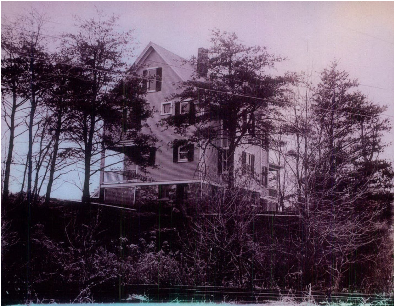
Figure 2: View of the Reynolds House, looking at the north (rear) and west (side) elevations from the former Glen Echo Railroad line, ca. 1900. The track is visible in the foreground. Source: Wooden Family Archives.
