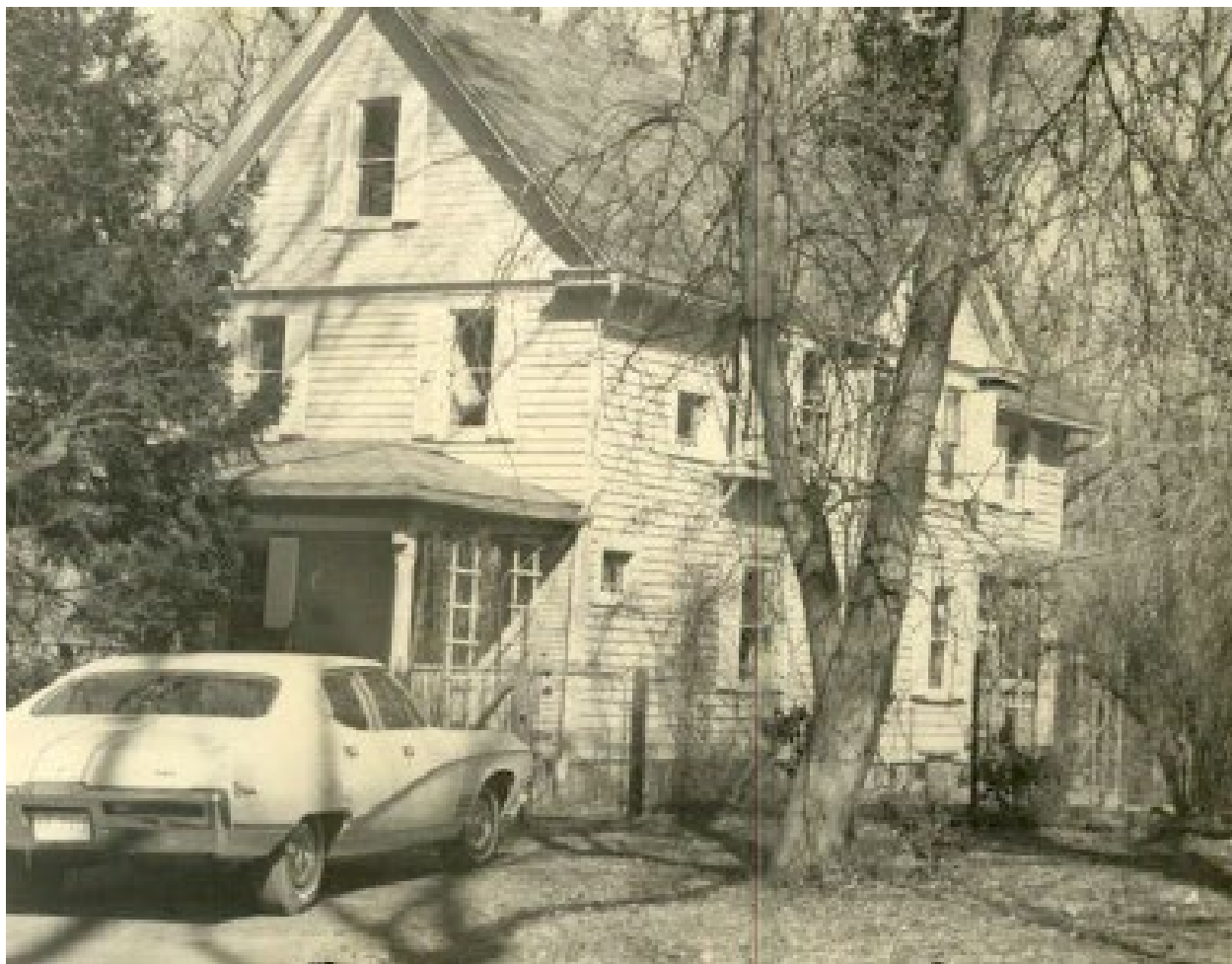
Figure 5: View of the Reynolds House, looking at the south (front) and east (side) elevations, 1970. Source: Montgomery County Parks.
