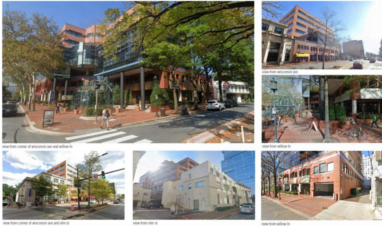
Figure 2: Existing conditions of the Property. The existing building consists primarily of brick with relatively uniform fenestration around the building aside from some variation on the southwest corner.
