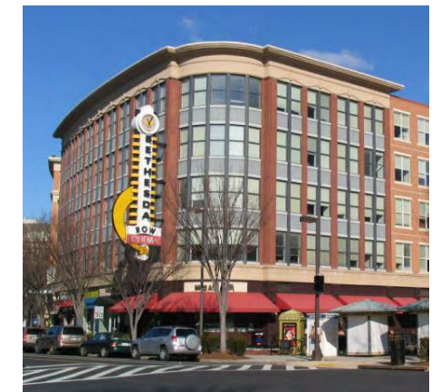
The curved corner along this major Bethesda Row intersection enhances pedestrian flow and provides an active ground floor.
