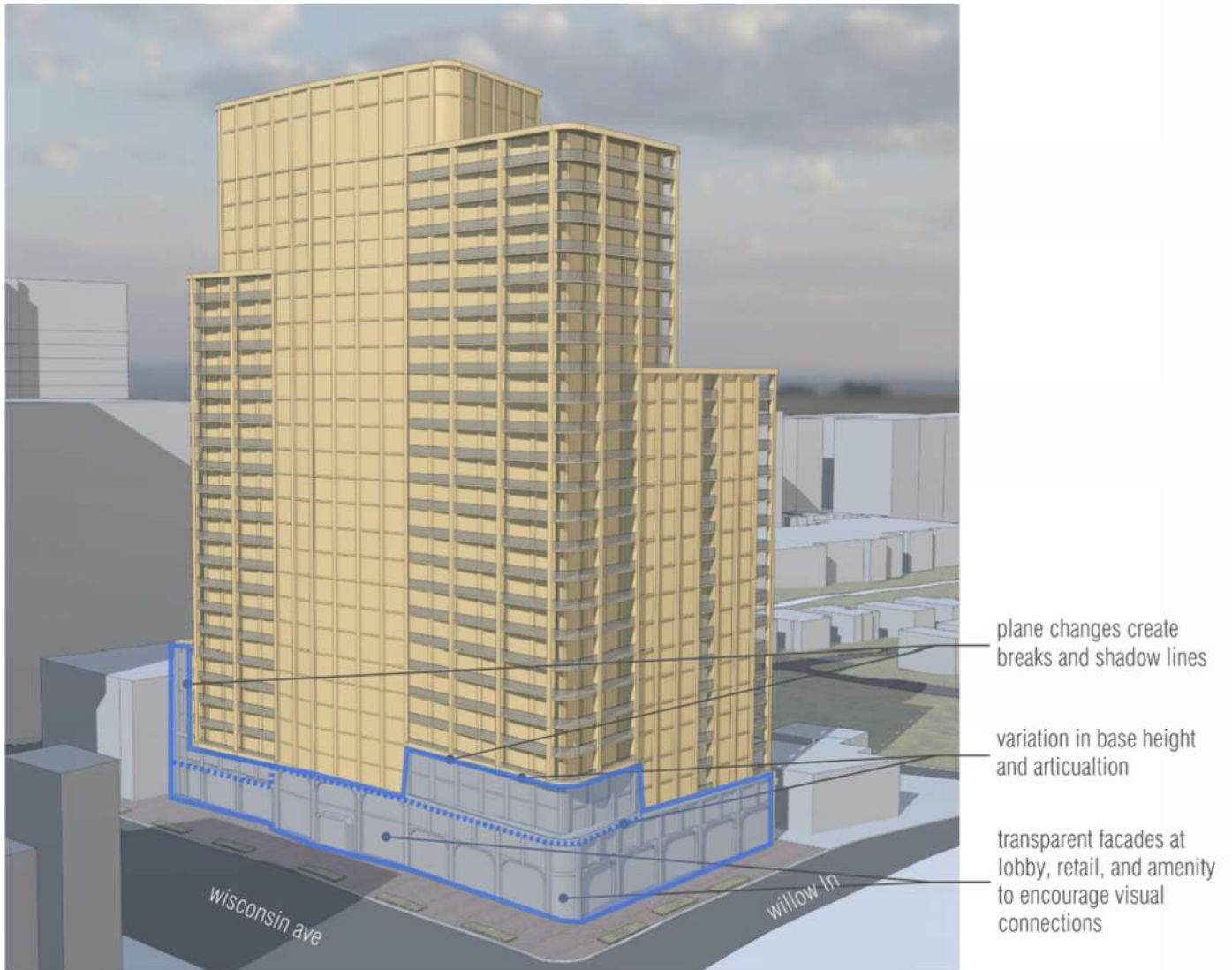
Figure 5: Proposed rendering showcasing Wisconsin Avenue and Willow Lane frontages. The Project will reactivate the Wisconsin and Willow Lane streetscapes with attractive retail and residential amenity space, plus adaptively reuse the existing underground parking garage for residents and retail visitors.
