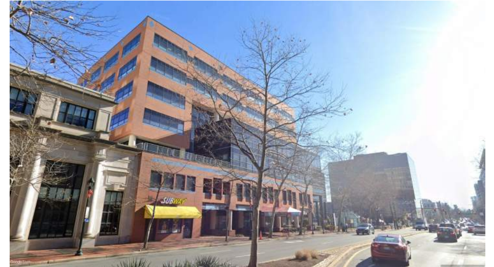
view from wisconsin ave
