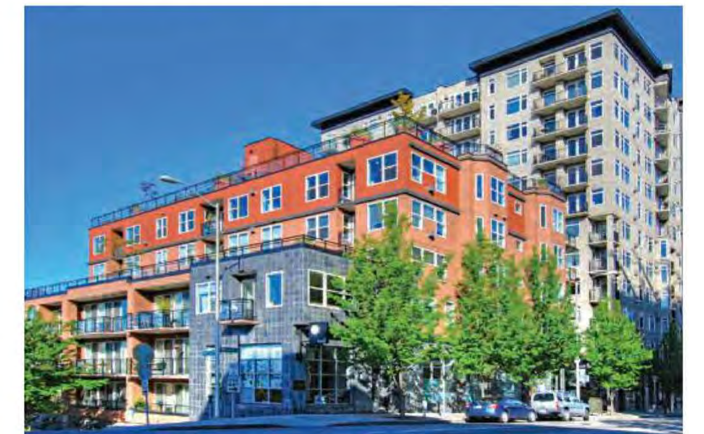
Transitions from Wisconsin Avenue to surrounding neighborhoods require stepping down of buildings to mediate between the high-rise and low-rise scales of the two areas. Source: The Vine Condos
