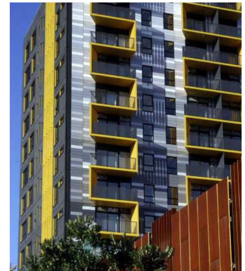
Balconies provide shadows and limit reflections on glass to deter birds. Source: Merchant Quarter Condominiums
