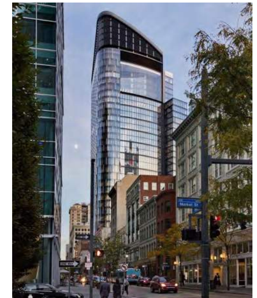
The form of the tower top for this Pittsburgh office building is part of the energy efficient solar chimney design. Source: Gensler
