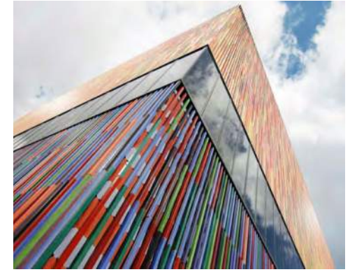
Patterns on this glass building reduce the likelihood of bird collisions. Source: naturalimages.net
