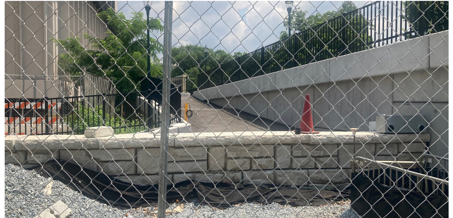
2. BOTTOM OF RAMP
