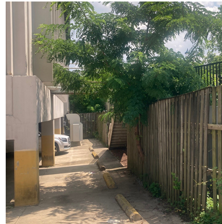
4. BOTTOM OF EXISTING OFFICE BUILDING
