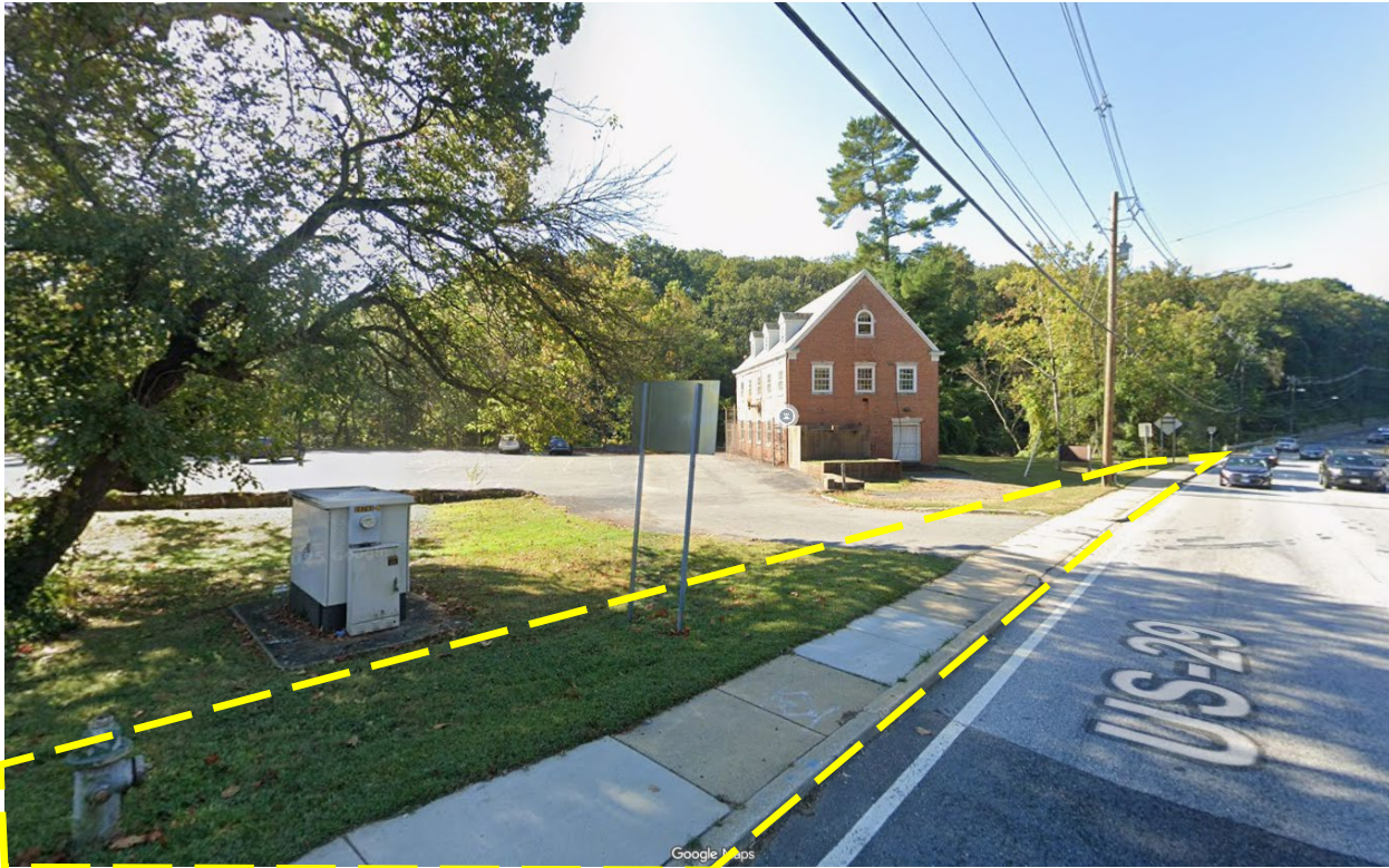
View southwest of former high lift pumping station within Burnt Mills East Park, showing extent of limits of grading within area of yellow dashed line.
