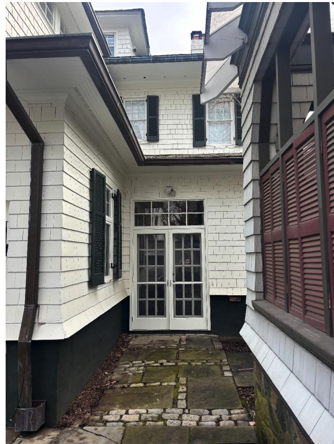
Existing Rear Entry
