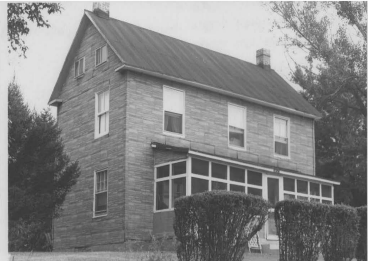
Figure 20: Rose Budd Home with asphalt as siding. Source: Maryland Historical Trust Worksheet, Montgomery Planning.
