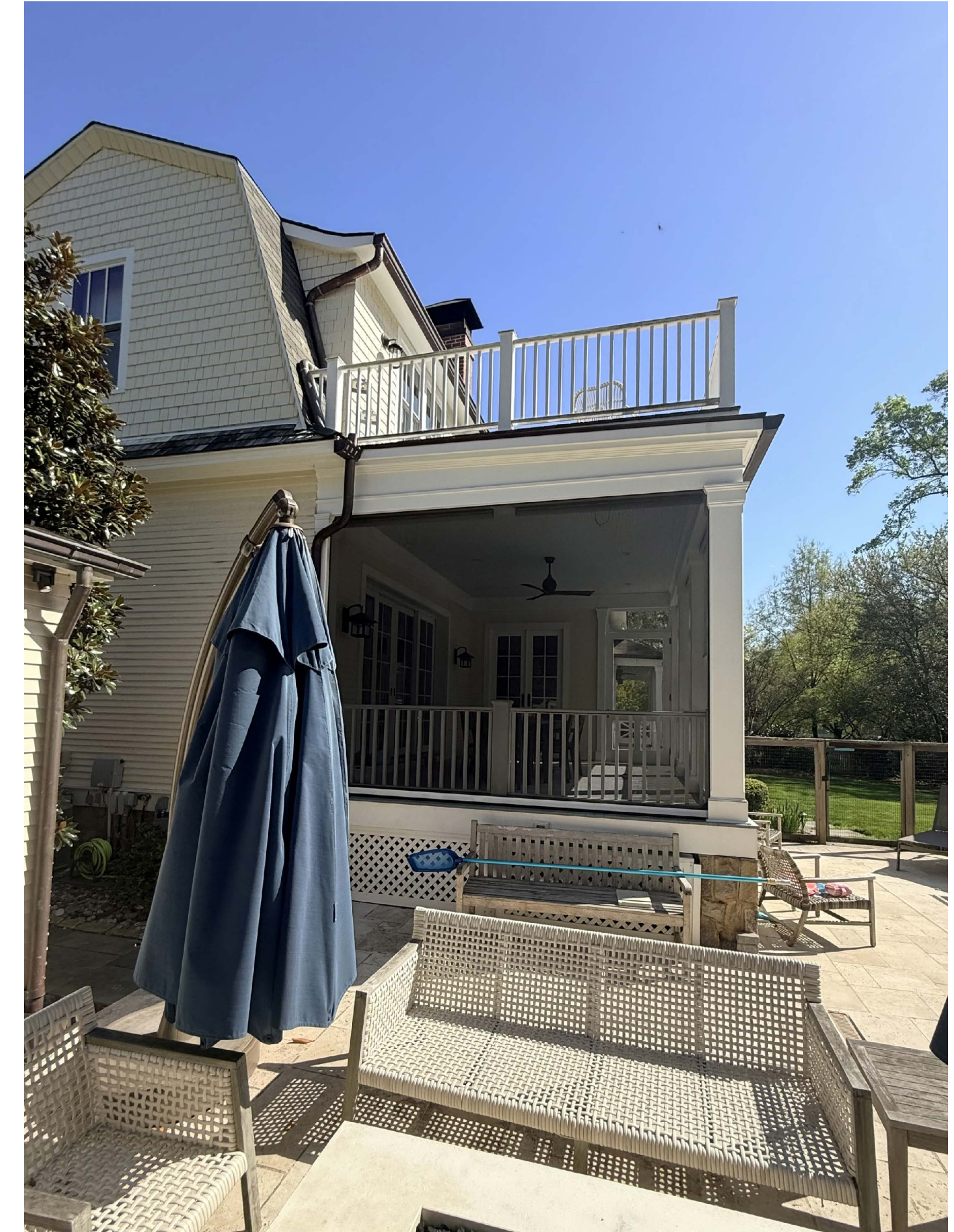
5 VIEW OF EXISTING SCREEN PORCH W/ DECK ABOVE A503 SCALE: N/A
