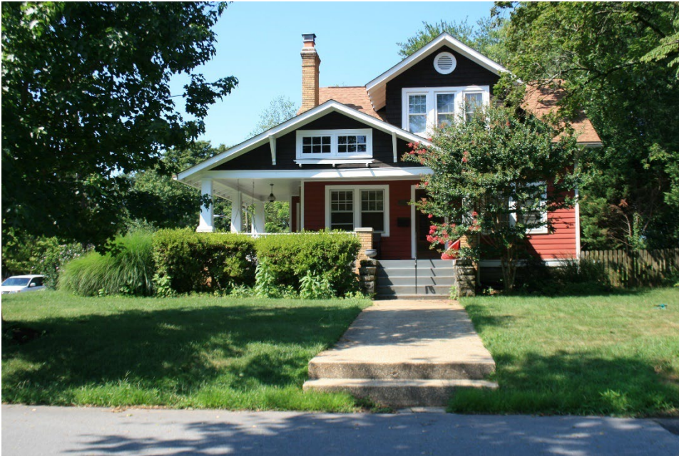
Figure 22: View of the Wilbur and Nellie Parsley House at 8800 First Avenue, 2020. Source: Montgomery Planning.
