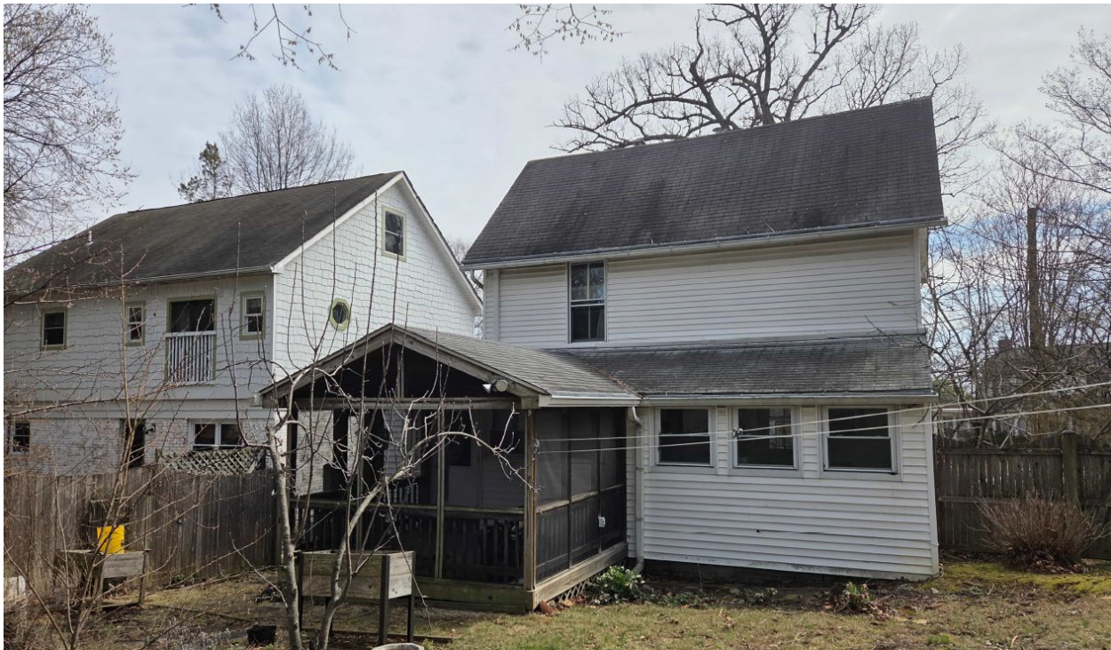
Figure 11: Rear view of subject property (Applicant).
