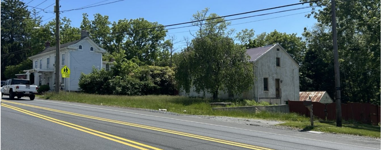
Figure 8: View southeast toward the subject property and adjacent historic property (May 2026, Historic Preservation Division).
