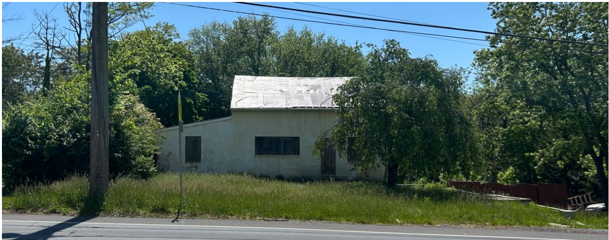
Figure 2: View of the subject property from Frederick Road (May 2026, Historic Preservation Division).
