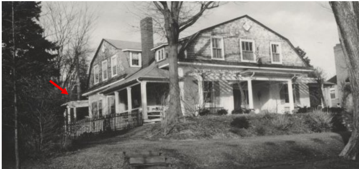
Figure 4: Circa 1993 photograph of the subject property from Grafton Street (Source: David Orem, Chevy Chase Historical Society). The proposed addition would be located over the pergola projecting on the far rear left in this photograph.
