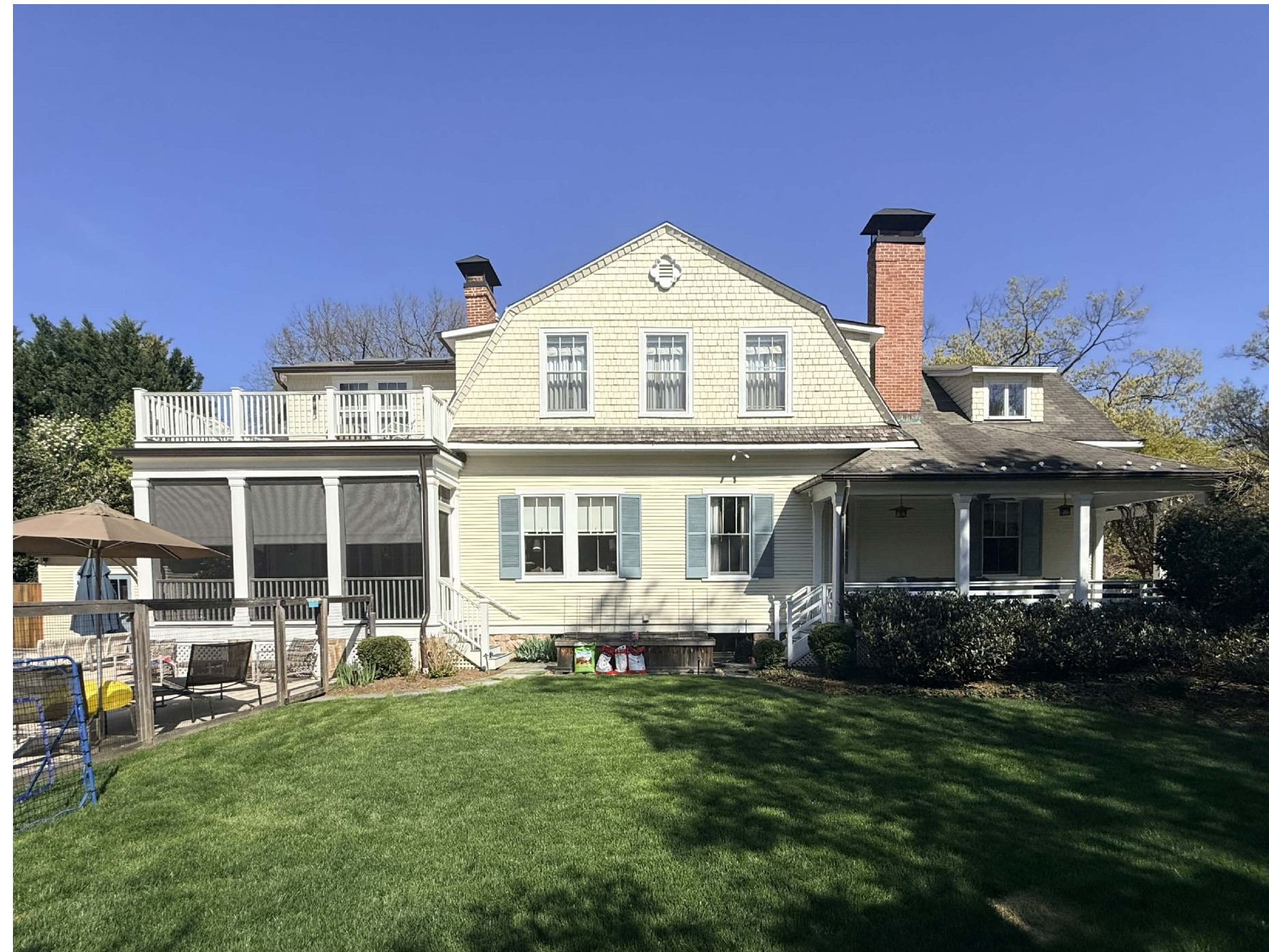
4 VIEW OF EXISTING RESIDENCE FROM WEST A503 SCALE: N/A
