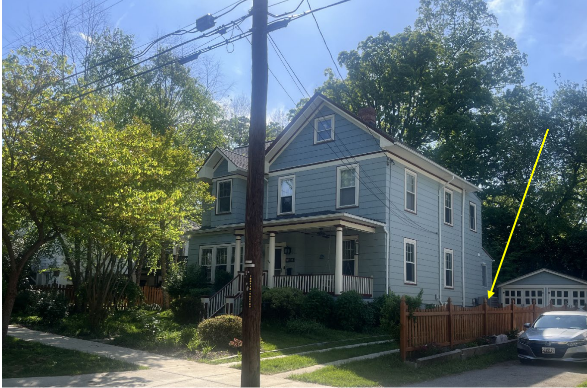
Figure 7: View of subject property from Spruce Avenue. Location of new stoop is annotated with a yellow arrow.
