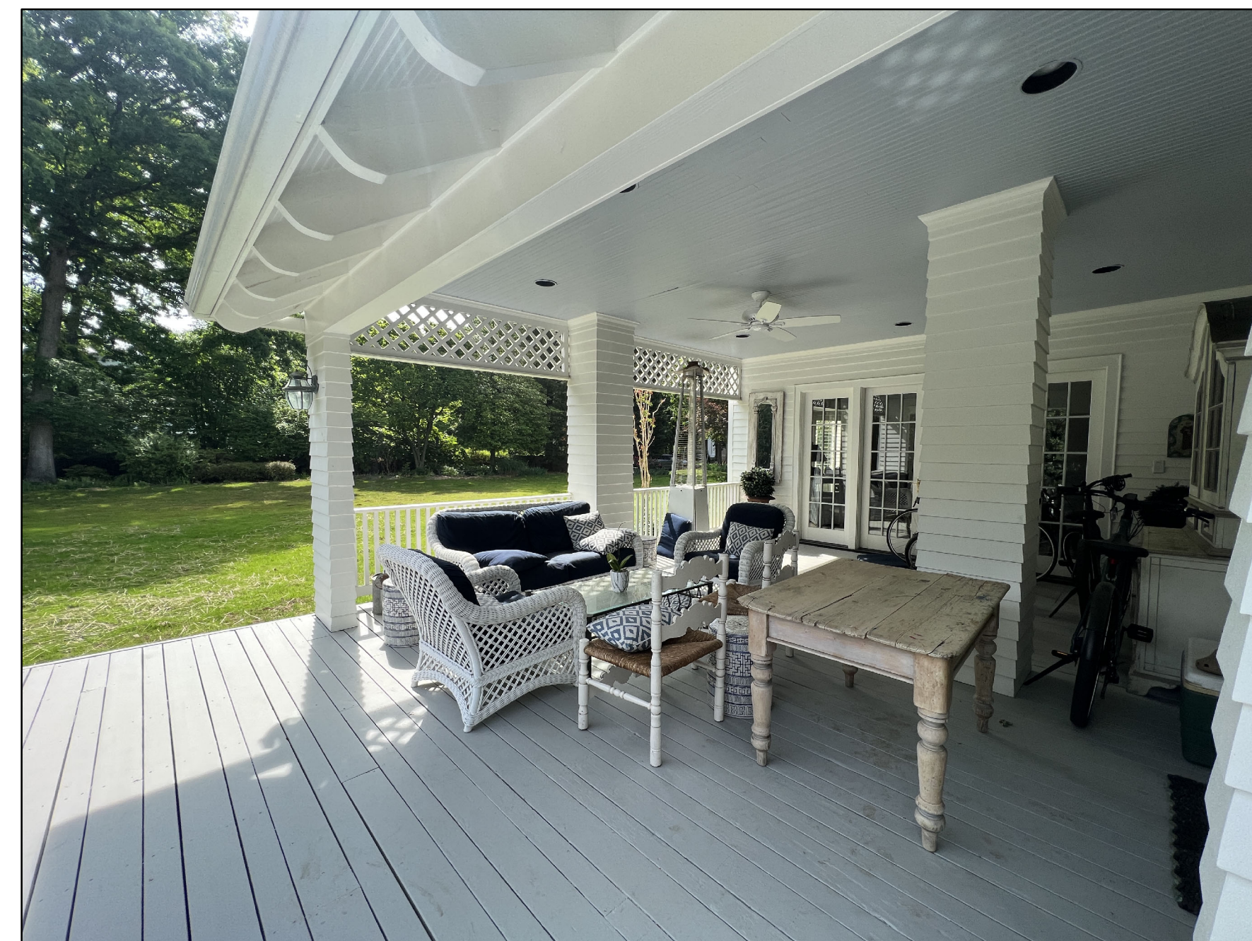
B2 A12 EXISTING EXTERIOR VIEW - REAR PORCH NT6
