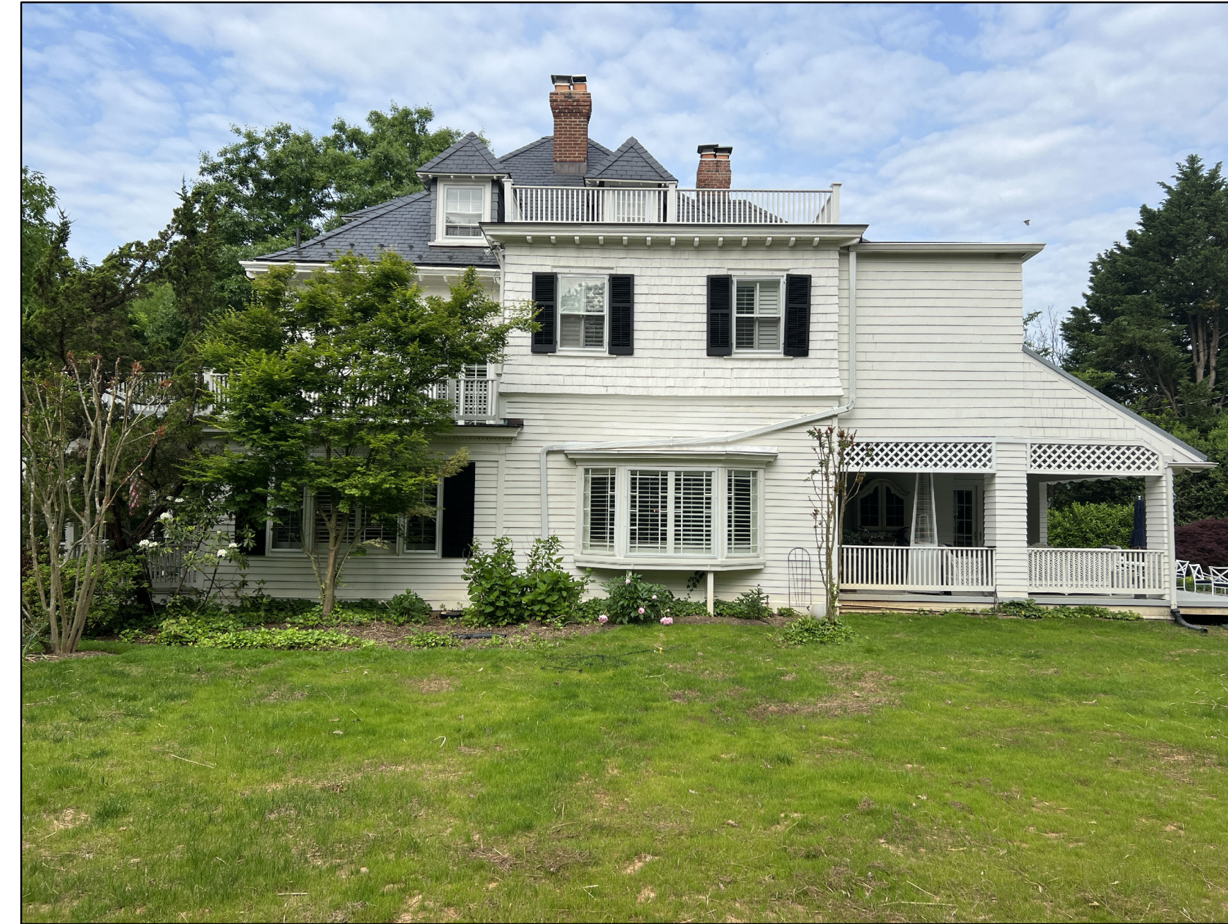
A2 A12 EXISTING EXTERIOR VIEW - WEST NT6
