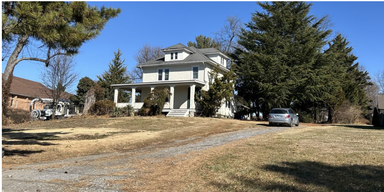
Figure 2: View of the subject property from Davis Mill Road (January 2026, Historic Preservation Division).
