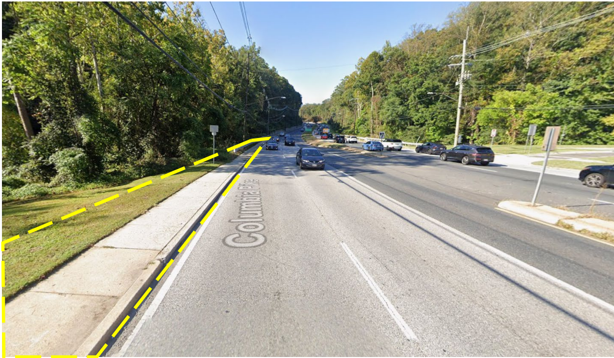
View southwest, south of former high lift pumping station within Burnt Mills East Park, showing extent of limits of grading within area of yellow dashed line.
