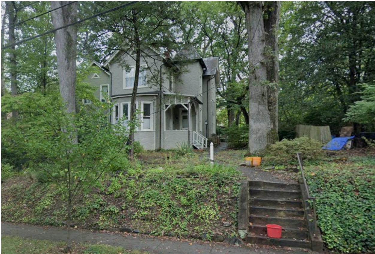
Figure 2: The subject property with the stairs and walkway to be replaced to the right.
