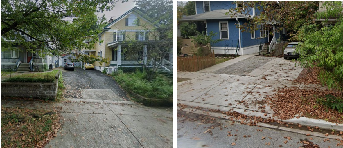
Figure 4: Driveways at 505 Tulip Avenue (left) and 502 Tulip Avenue (right).
