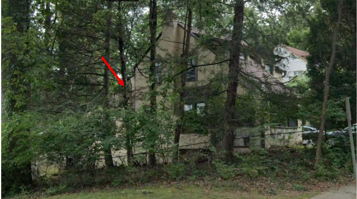
Figure 3: View from Philadelphia Avenue towards the location of the proposed enclosure (marked with a red arrow) at the rear of the house.
