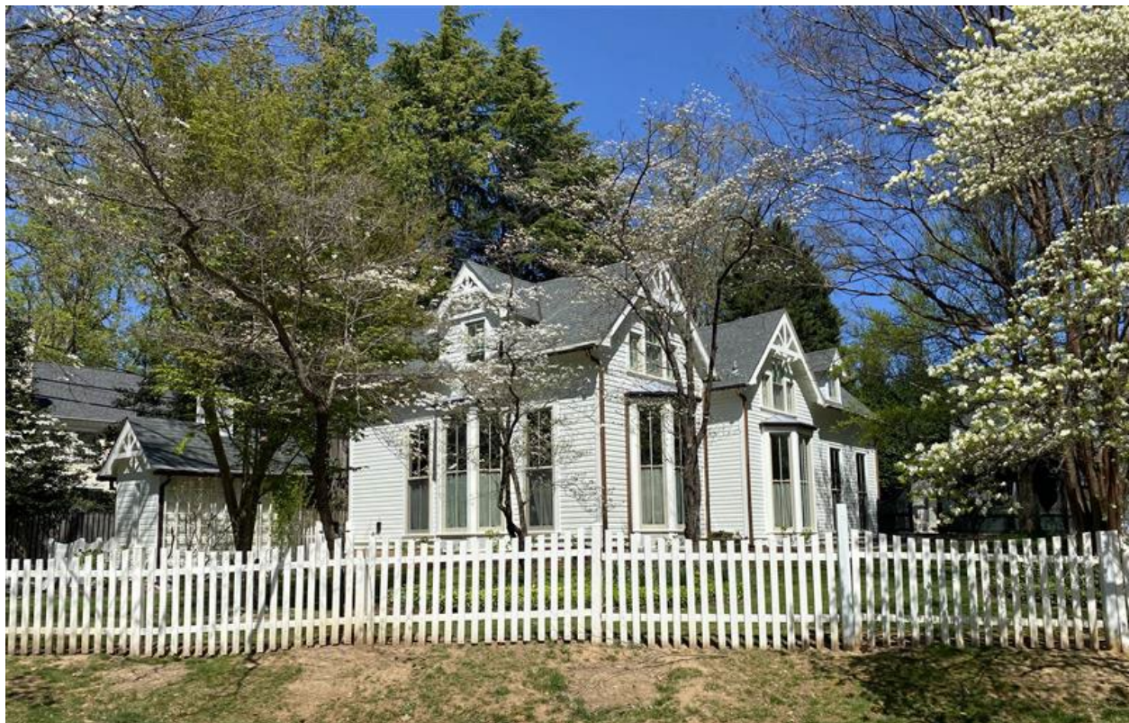
Figure 2: The facade and left elevation of the property from Magnolia Avenue.
