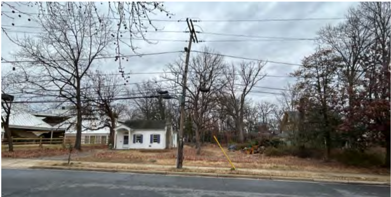
Figure 2: Front and partial side elevation of the existing Non-Contributing house at 707 New York Avenue, with the neighboring Outstanding resource on the adjacent parcel at 703 Takoma Avenue visible on the far right (December 2025, Historic Preservation Division).
