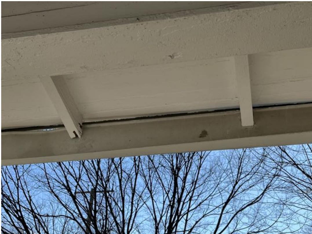
Detail: 6704 WESTMORELAND AVE. PORCH ROOF RAFTERS
