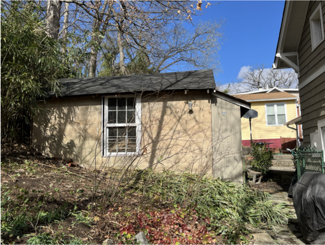
Detail: 6704 WESTMORELAND AVE. SHED (EAST-FACE)
