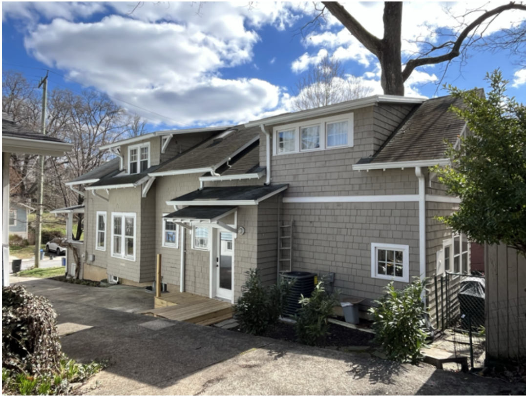
Detail: 6704 WESTMORELAND AVE. (SOUTH-WEST) CORNER
