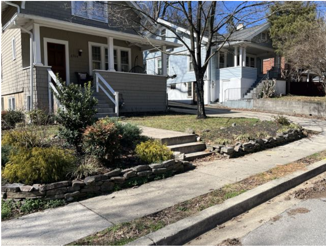
Detail: 6704 WESTMORELAND AVE. LOW STONE WALLS
