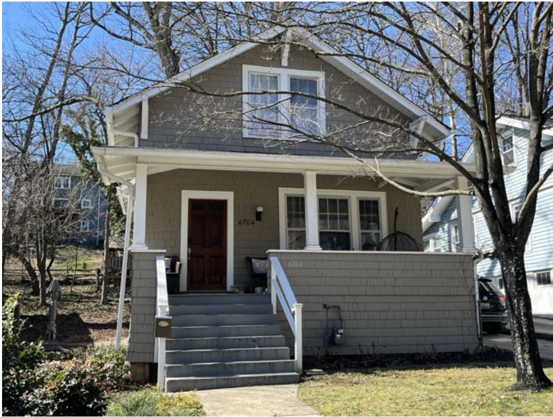
Detail: 6704 WESTMORELAND AVE.(NORTH) FRONT
