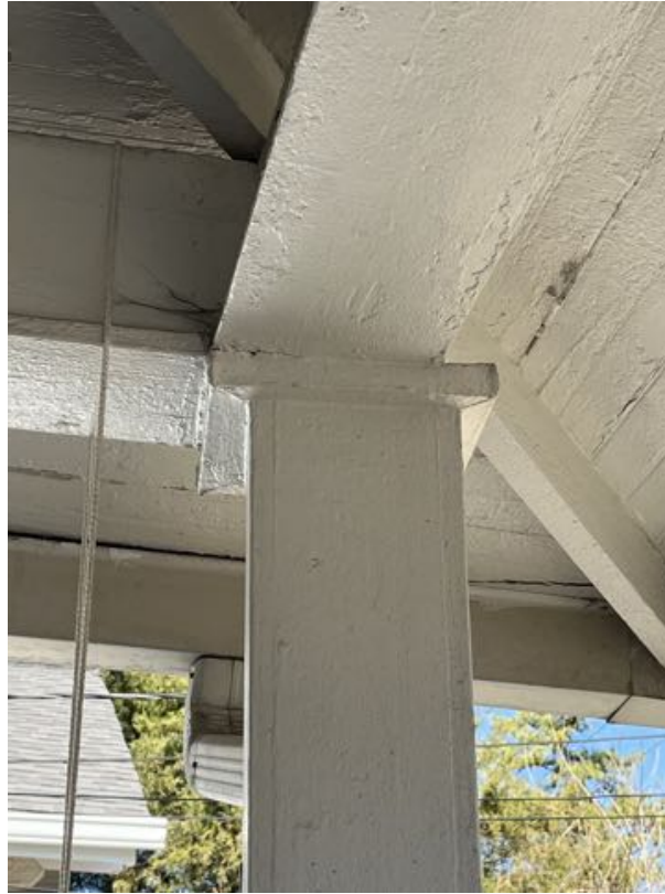
Detail: 6704 WESTMORELAND AVE. PORCH COLUMN CAP
