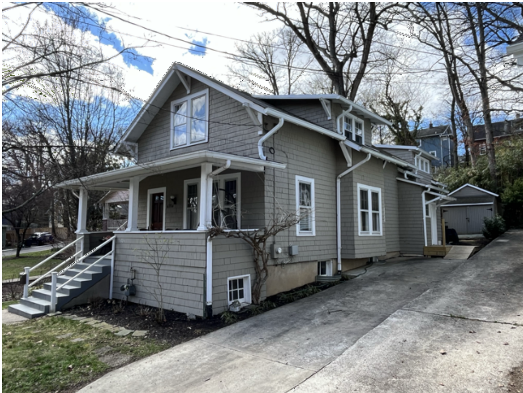
Detail: 6704 WESTMORELAND AVE.(NORTH-WEST) CORNER.
