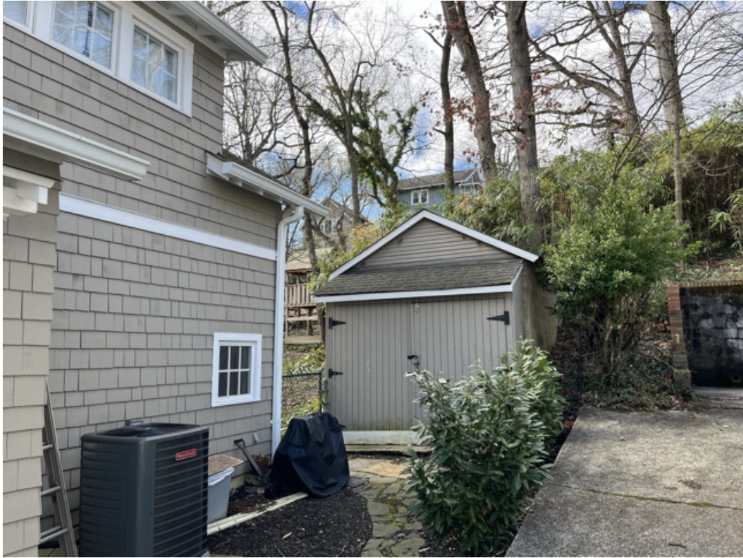
Detail: 6704 WESTMORELAND AVE. SHED
