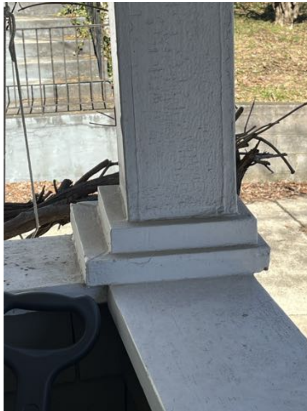
Detail: 6704 WESTMORELAND AVE. PORCH COLUMN BASE
