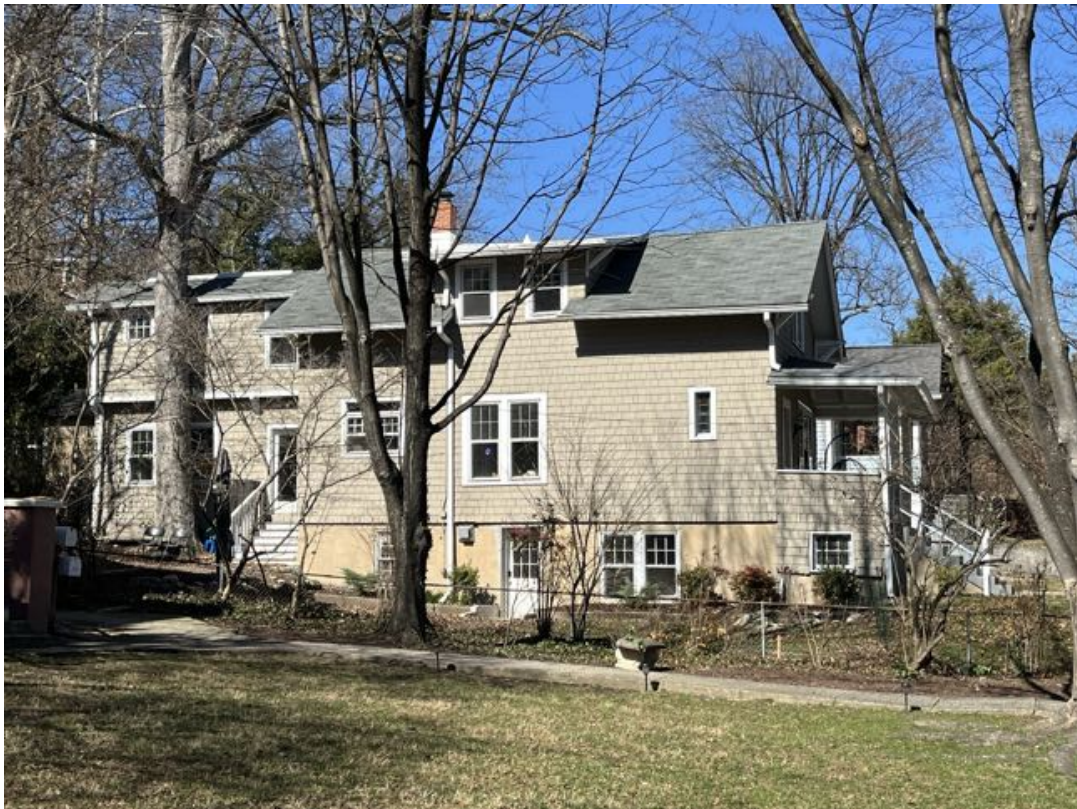
Detail: 6704 WESTMORELAND AVE. (EAST) SIDE
