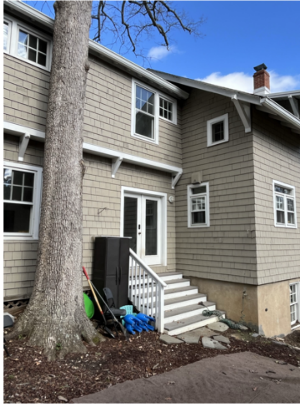
Detail: 6704 WESTMORELAND AVE. (SOUTH-EAST) FAMILY ROOM ENTRY
