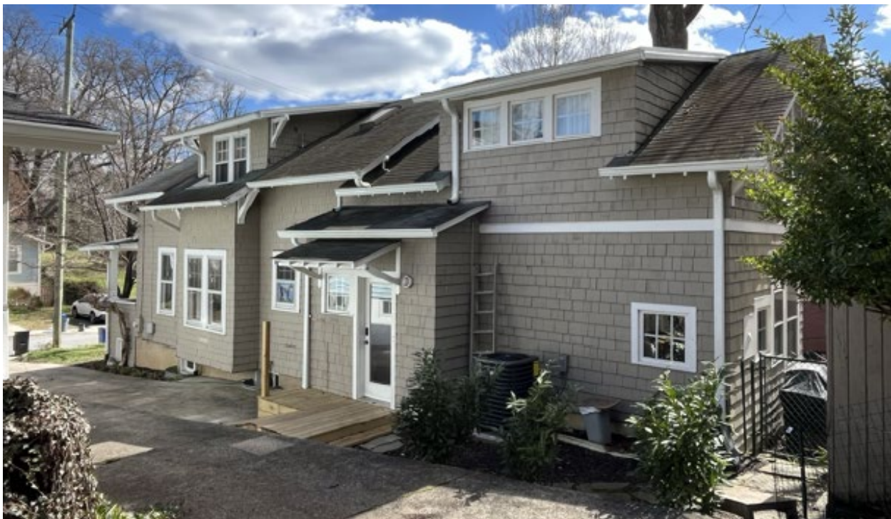
Figure 5: Existing northwest side elevation photograph.
