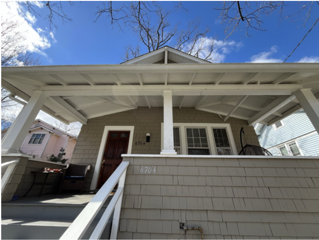
Detail: 6704 WESTMORELAND AVE. PORCH ROOF
