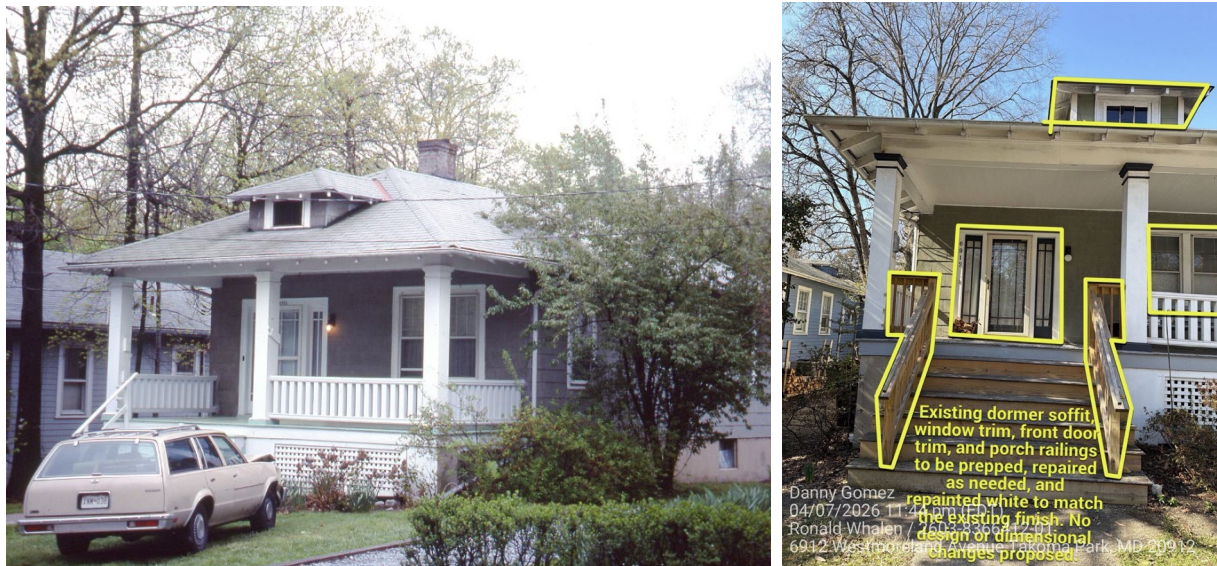
Figure 2: Photo of the subject property c. 1990 (left; Montgomery County Planning) and 2026 (right; Danny Gomez).
