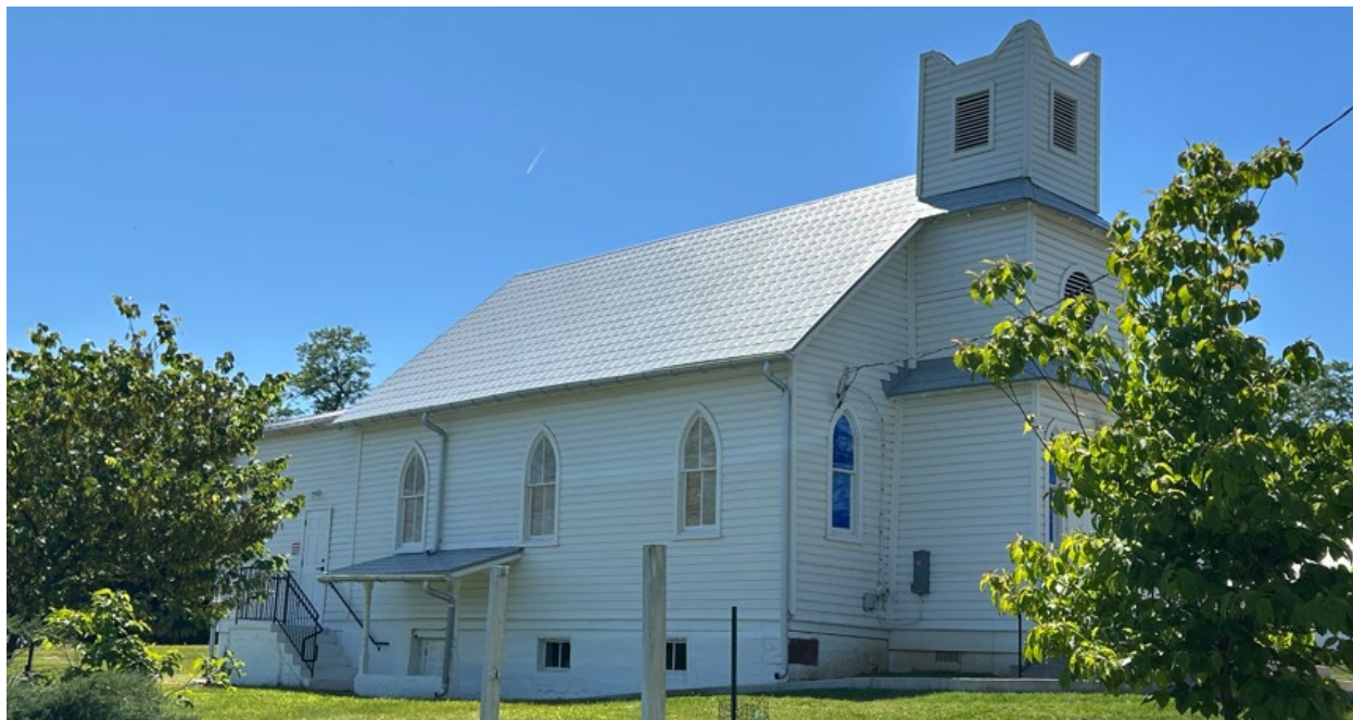
Figure 2: Existing front and southeast side elevation (May 2026, Historic Preservation Division).
