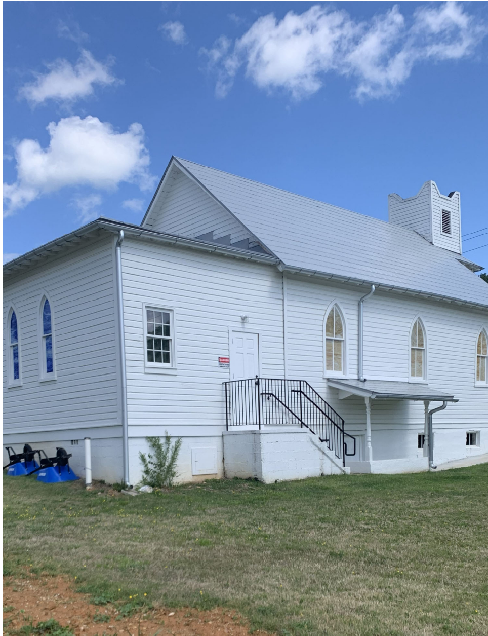
Photo 3 - Pleasant View United Methodist Church - East Elevation -04/30/2026
