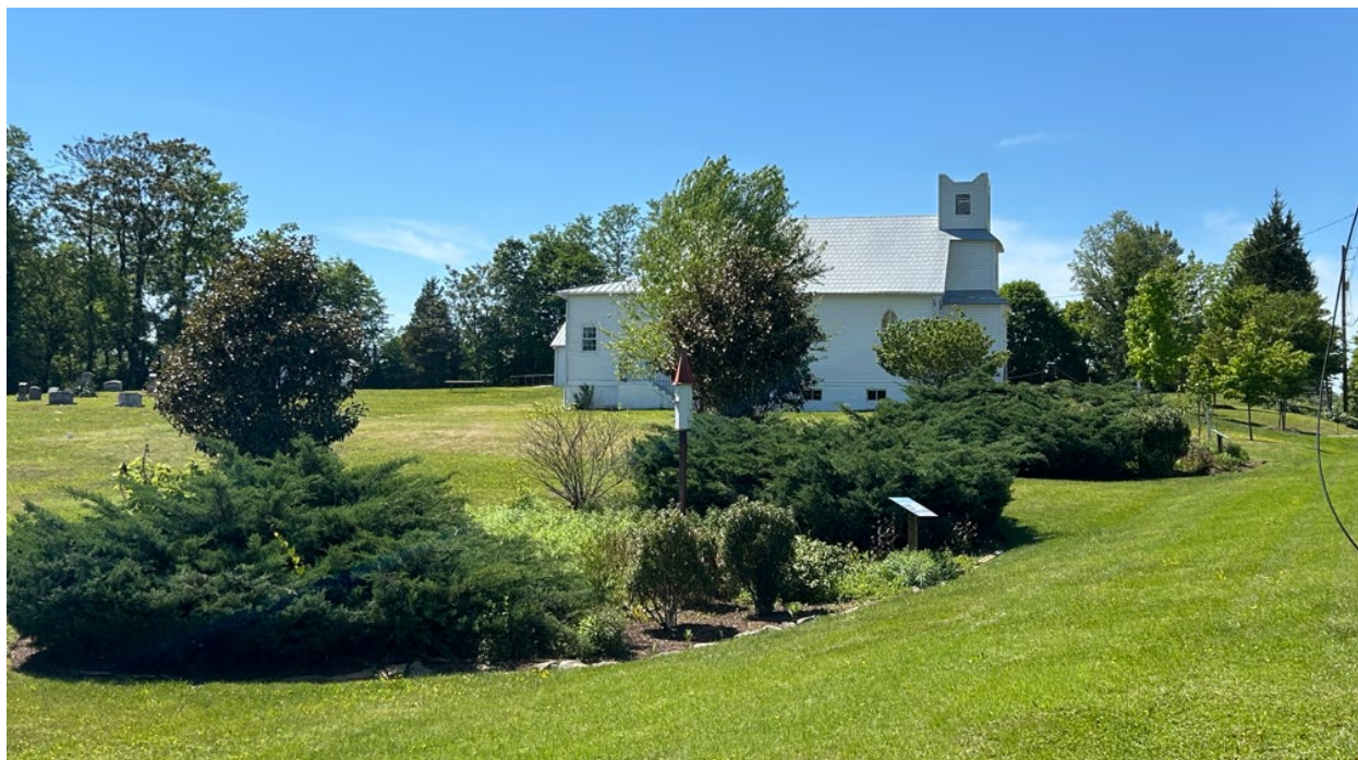
Figure 8: View towards the southeast side elevation of the subject property. The mechanical equipment at the rear of the structure may become visible at this distance, but would be screened behind new wood fencing.
