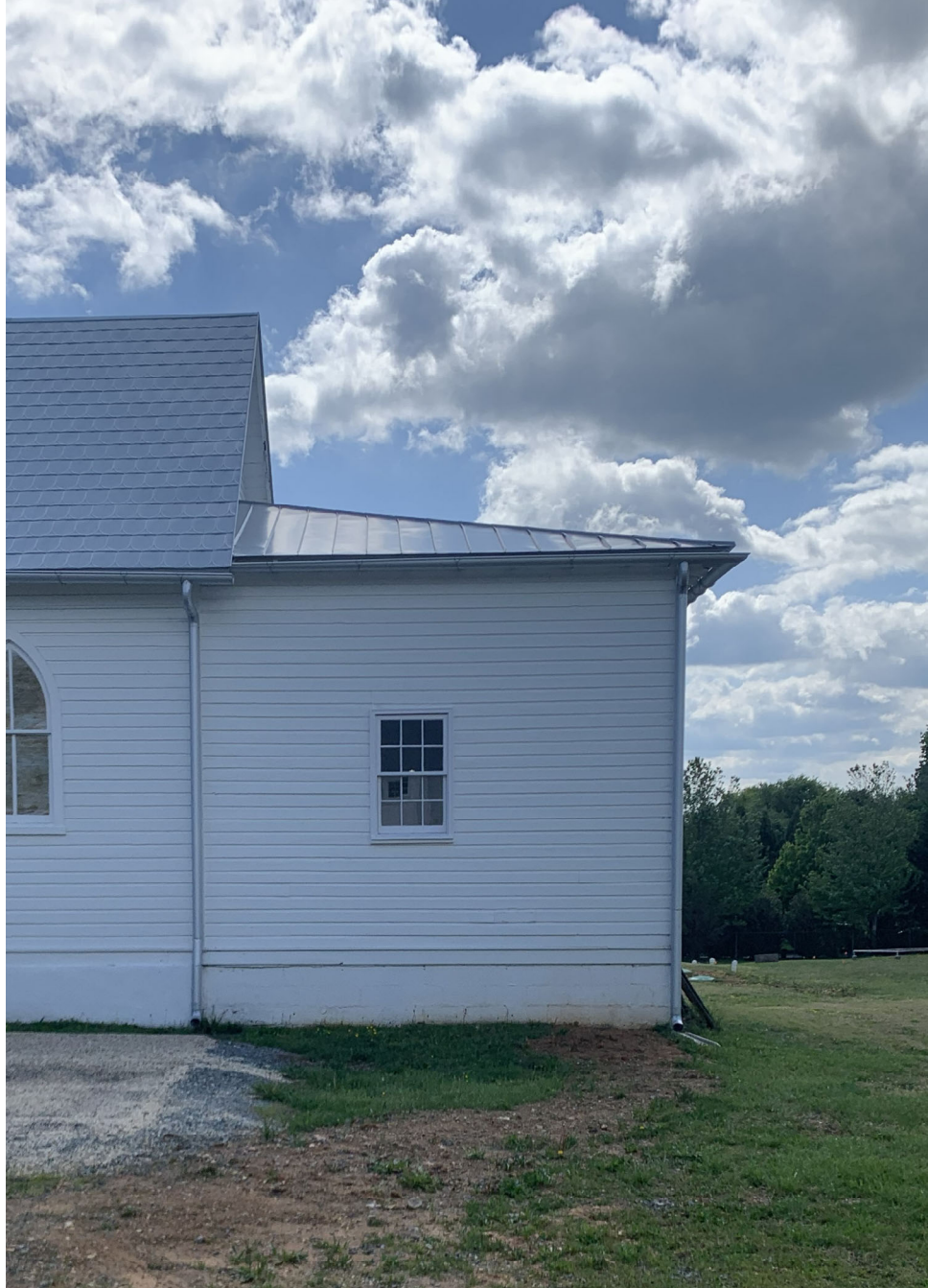
Photo 1- Pleasant View United Methodist Church - West Elevation -04/30/2026
