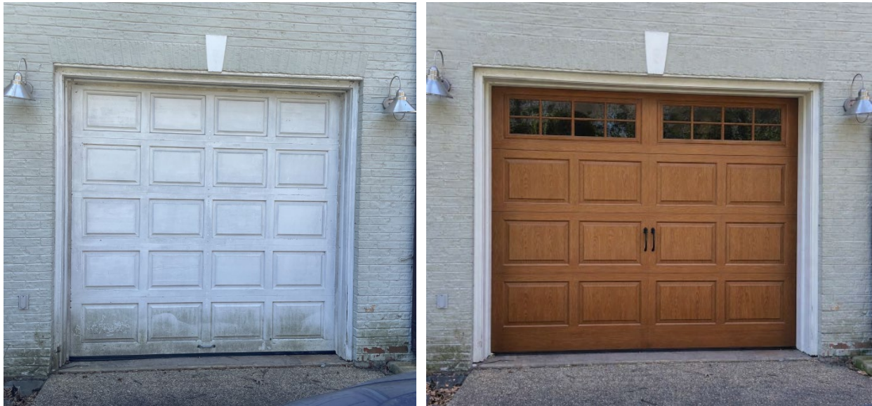
Figure 3: The existing garage door (left) and mock-up of the proposed steel door (right). Staff notes that the proposed door on the right appears wider than the existing door.
