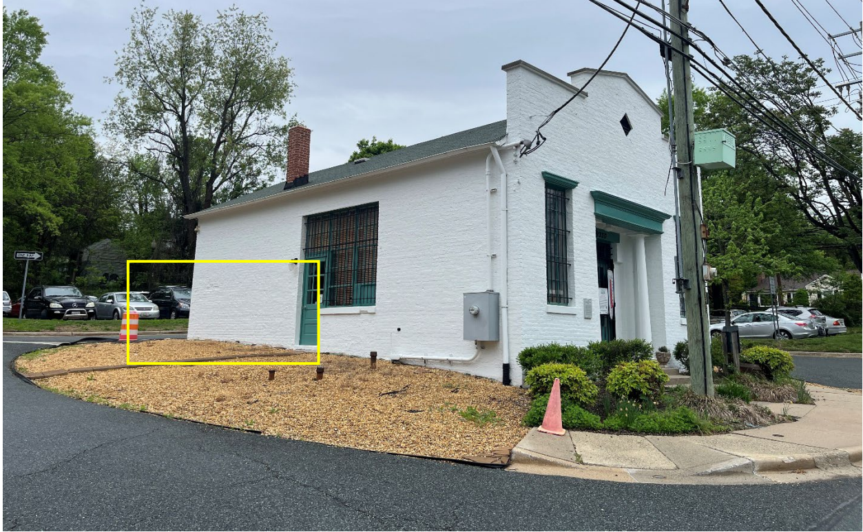
Figure 5: View of side elevation, with approximate location of ramp annotated with a yellow box.
