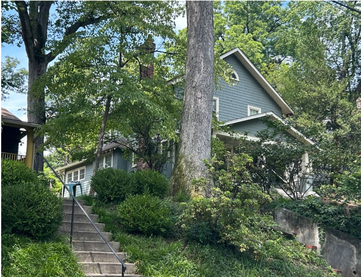
Figure 6: Southwest side elevation and southeast front elevation of the subject property showing visibility of the existing rear addition from the public right-of-way, August 2025 (Historic Preservation Office).
