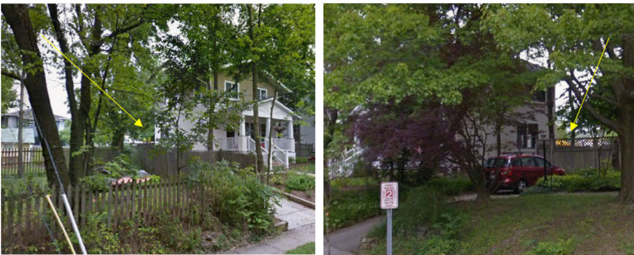
Figure 8: View of subject property from the right of way along Holt Place. The approximate location of the addition is indicated with a yellow arrow.
