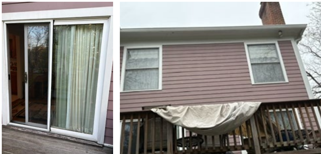
Figure 2: The existing patio doors (left) and windows (right) to be replaced.
