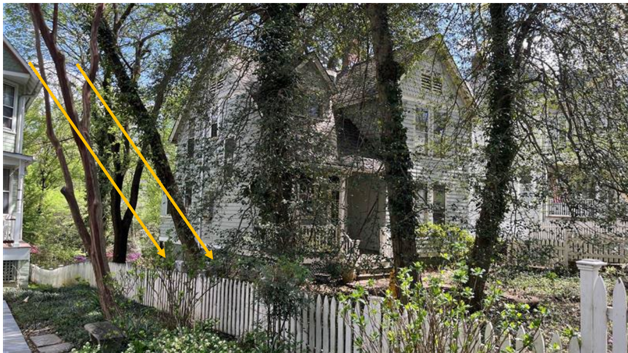
Figure 4: Approximate location of the units from the right-of-way.
