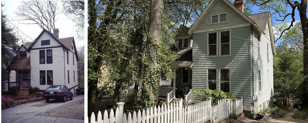
Figure 2: View of the subject property in c. 1990 (left) and 2026 (right). Both photos are courtesy of Montgomery County Planning Staff.
