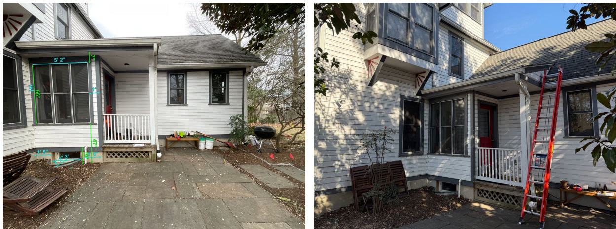
Figure 2: Existing rear of house, showing non-historic one-story addition
