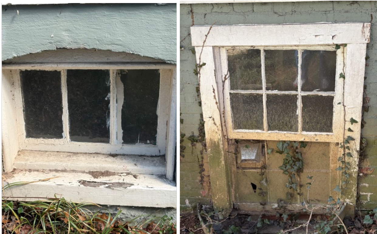
Figure 4: Foundation-level windows to be replaced.
