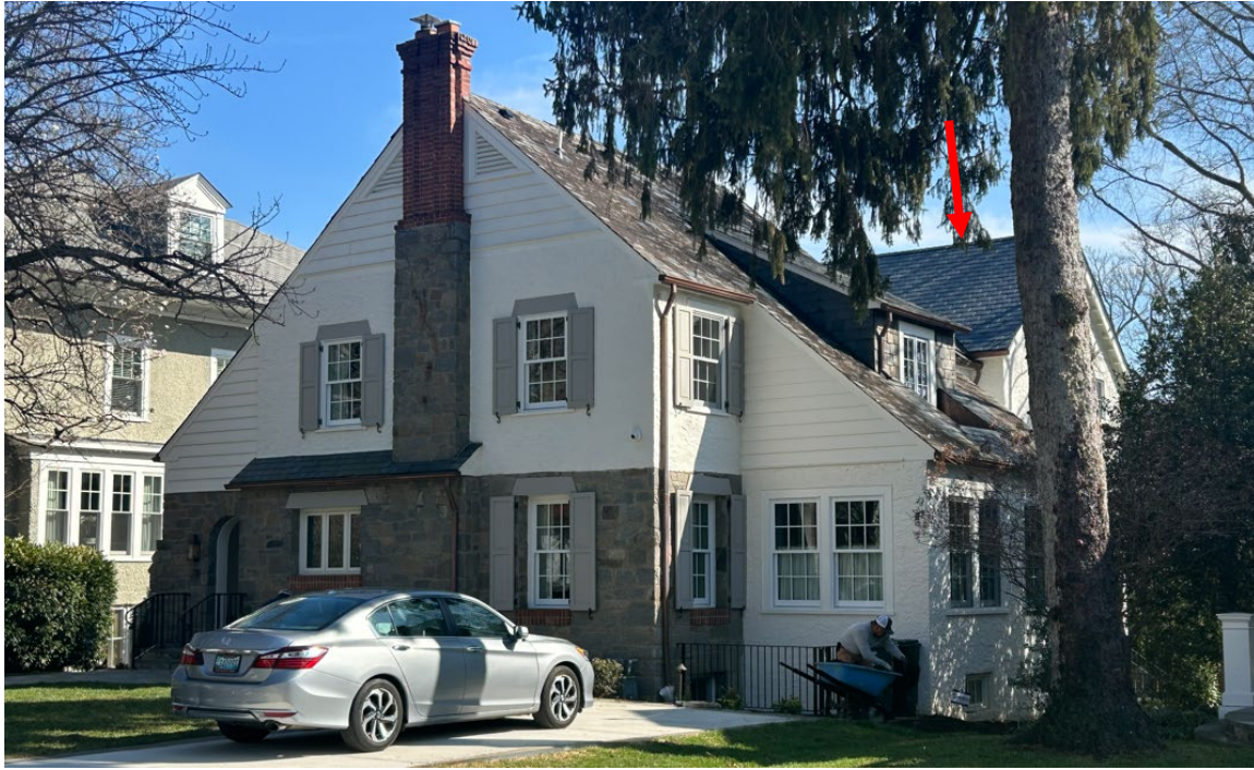
Figure 2: Front and partial west side elevation (March 2026, Historic Preservation Division). The existing slate on the main block would be replaced with synthetic slate to match that of the rear addition (shown with a red arrow).
