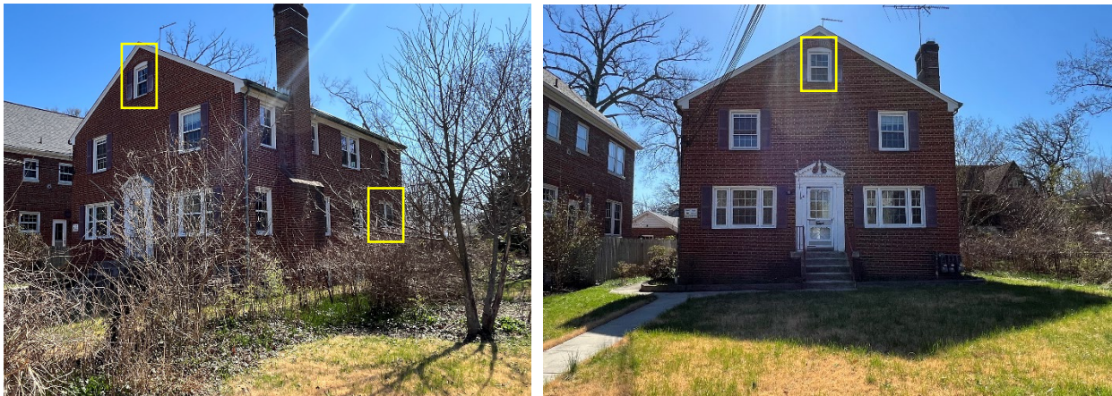
Figure 4: Window replacement visible from the right-of-way along Carroll Avenue are annotated with a yellow box.
