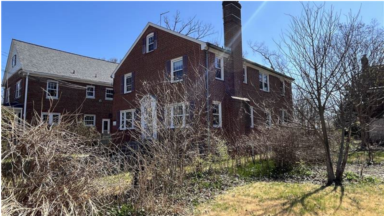
Figure 2: View of subject property from Carroll Avenue (Montgomery County Planning, 2026)
