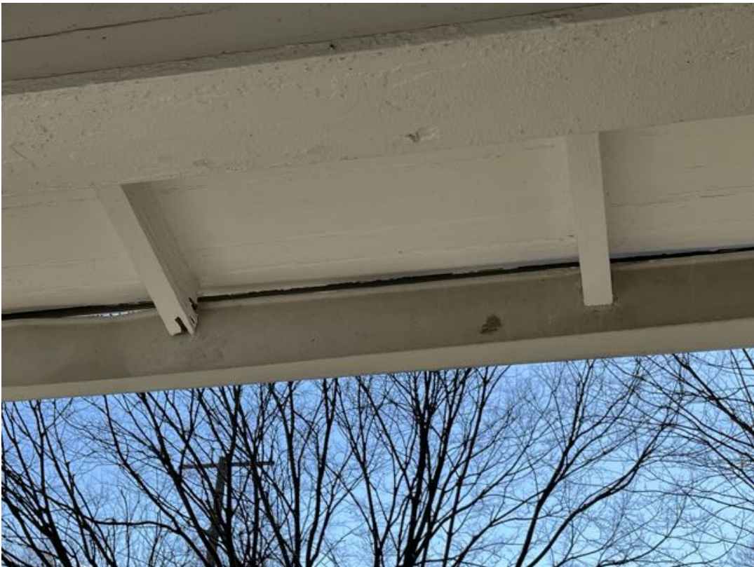
Detail: 6704 WESTMORELAND AVE. PORCH ROOF RAFTERS
