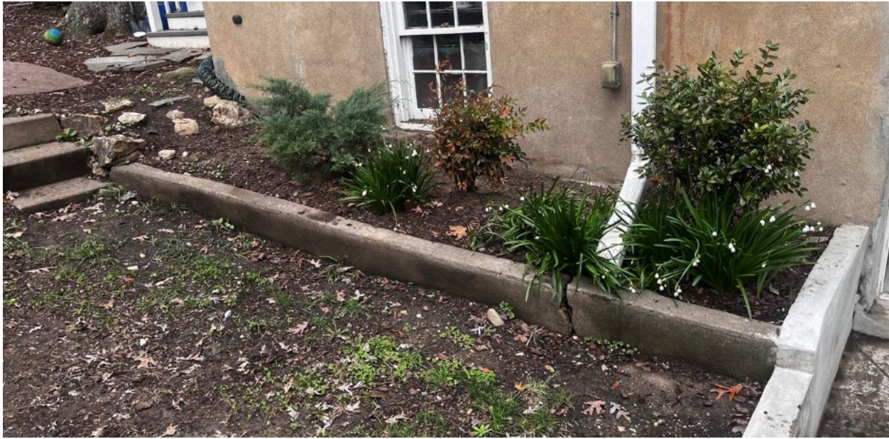
Figure 9: One of the concrete curbs to be removed.
