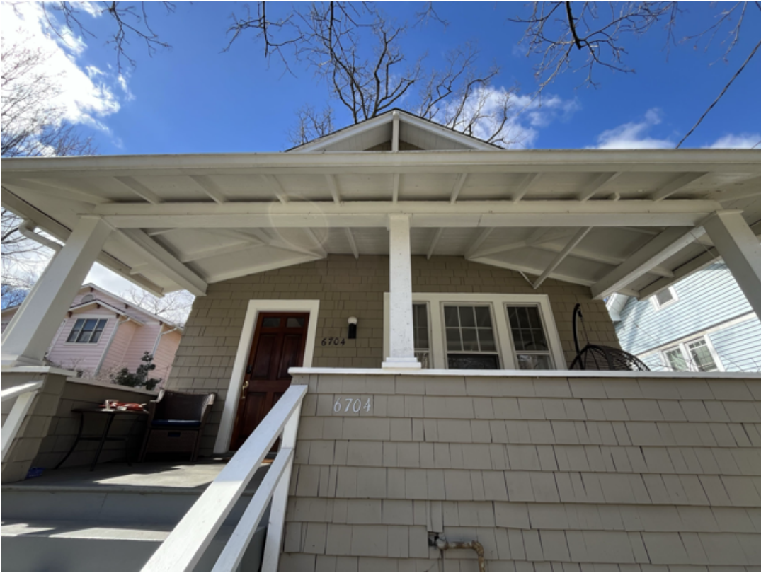
Detail: 6704 WESTMORELAND AVE. PORCH ROOF
