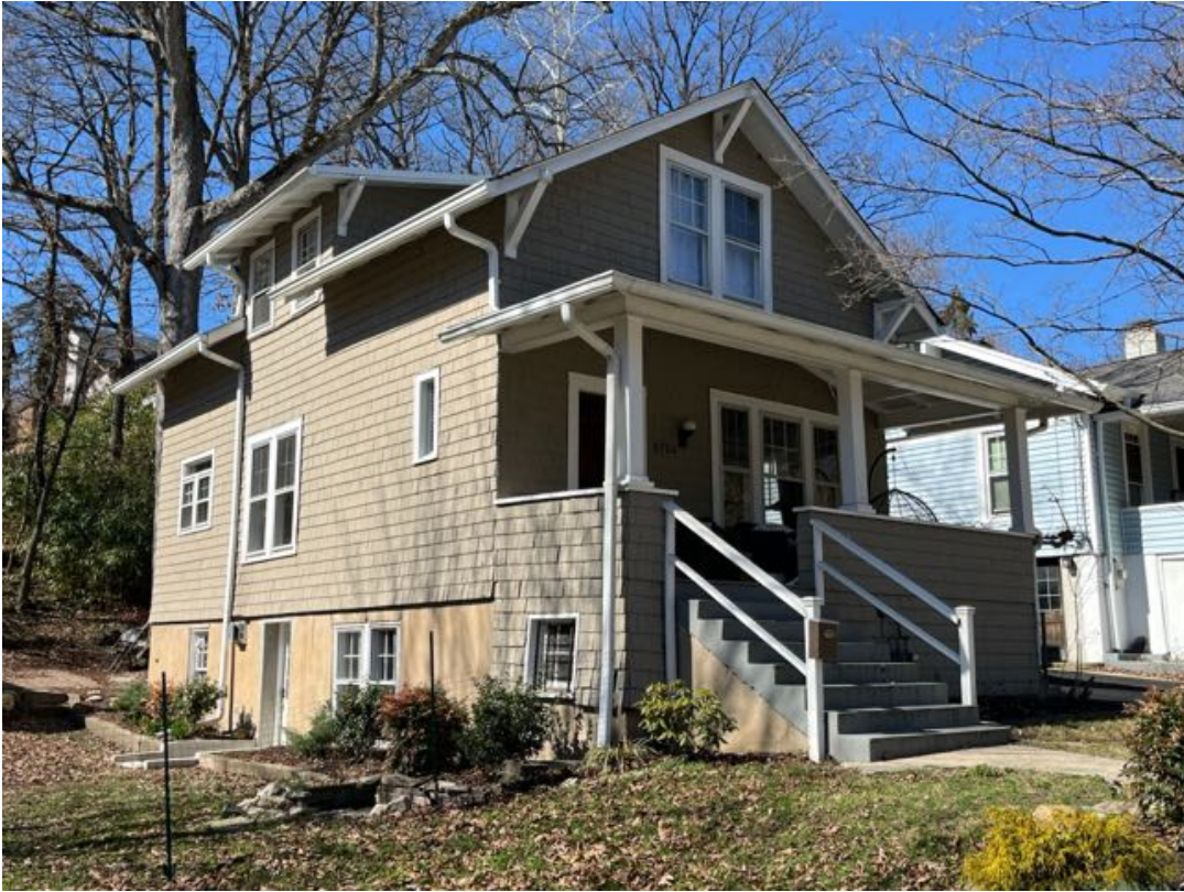
Detail: 6704 WESTMORELAND AVE. (NORTH-EAST) CORNER
