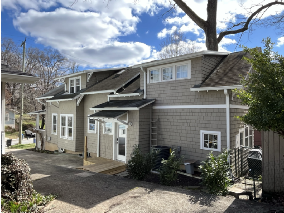
Detail: 6704 WESTMORELAND AVE. (SOUTH-WEST) CORNER
