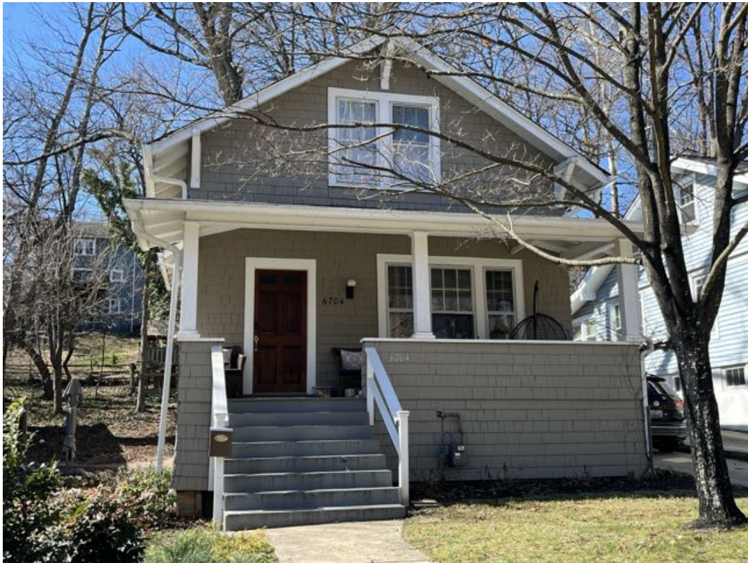
Detail: 6704 WESTMORELAND AVE.(NORTH) FRONT
