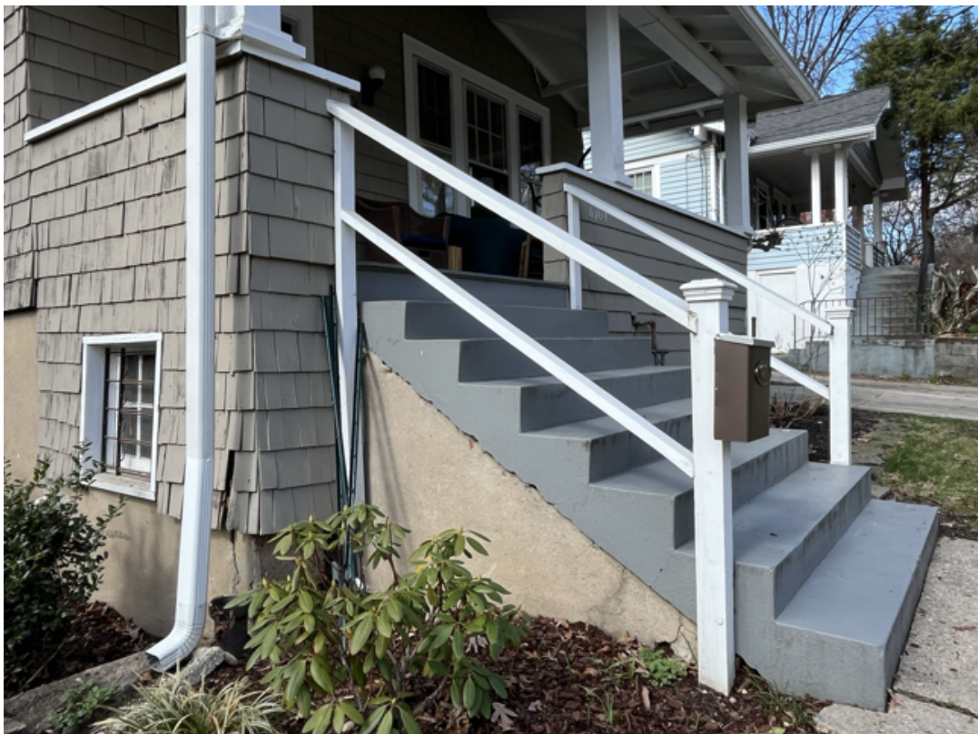
Detail: 6704 WESTMORELAND AVE. MASONRY PORCH STEPS
