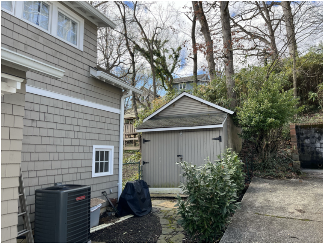
Detail: 6704 WESTMORELAND AVE. SHED
