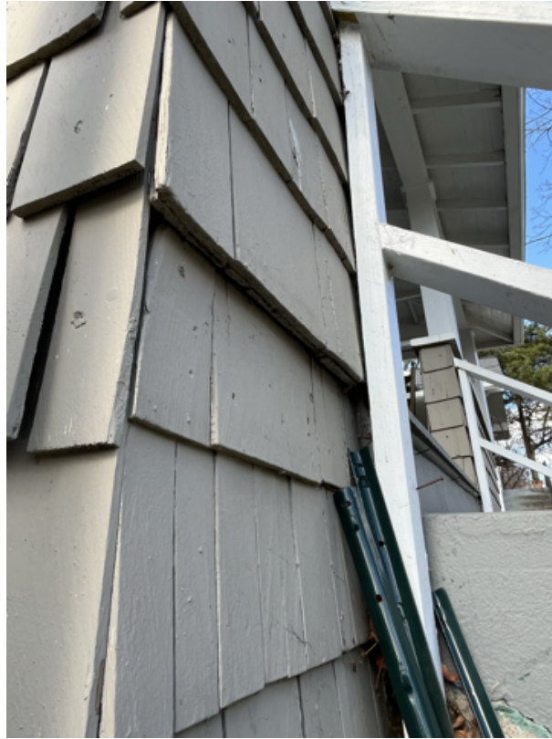
Detail: 6704 WESTMORELAND AVE. PORCH SIDING
