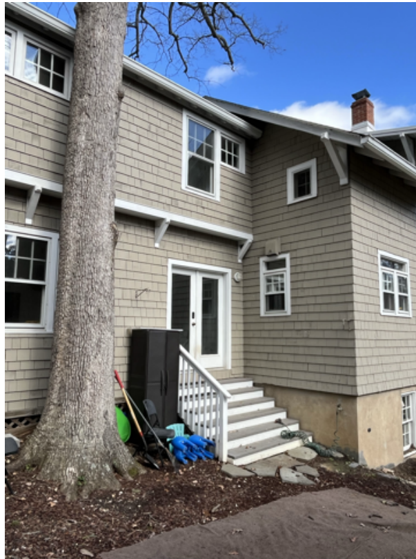
Detail: 6704 WESTMORELAND AVE. (SOUTH-EAST) FAMILY ROOM ENTRY
