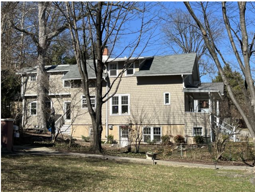
Detail: 6704 WESTMORELAND AVE. (EAST) SIDE
