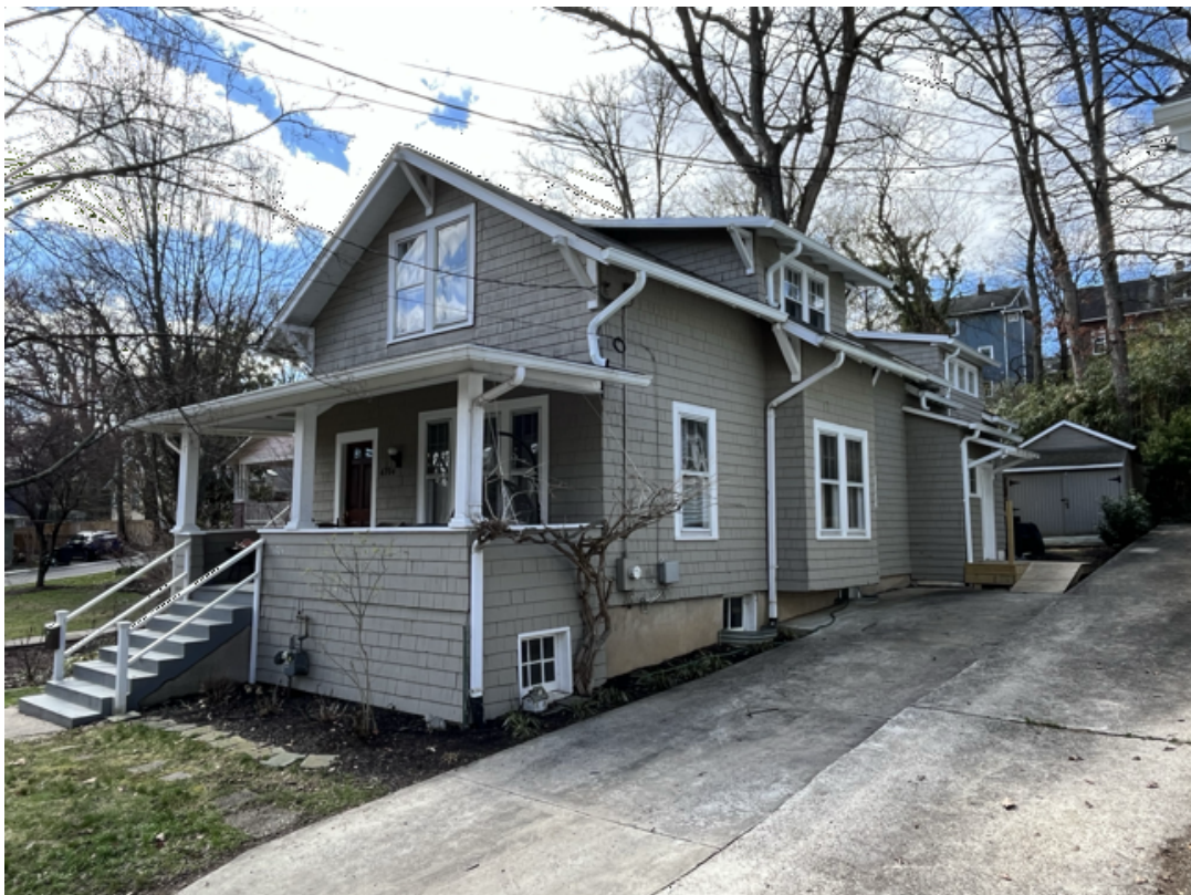
Detail: 6704 WESTMORELAND AVE.(NORTH-WEST) CORNER.
