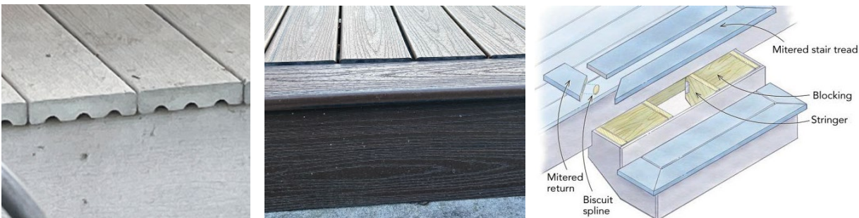
Figure 7: Edges of Trex decking (left), installation of edge boards (center), and installation of boards with mitered risers to obscured edges of stairs (right).
