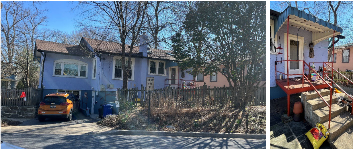
Figure 6: View of the west (rear) elevation and the metal landing (right).
