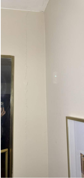
PHOTO 14: CRACKS IN EAST EXTERIOR WALL (UNIT 2)
