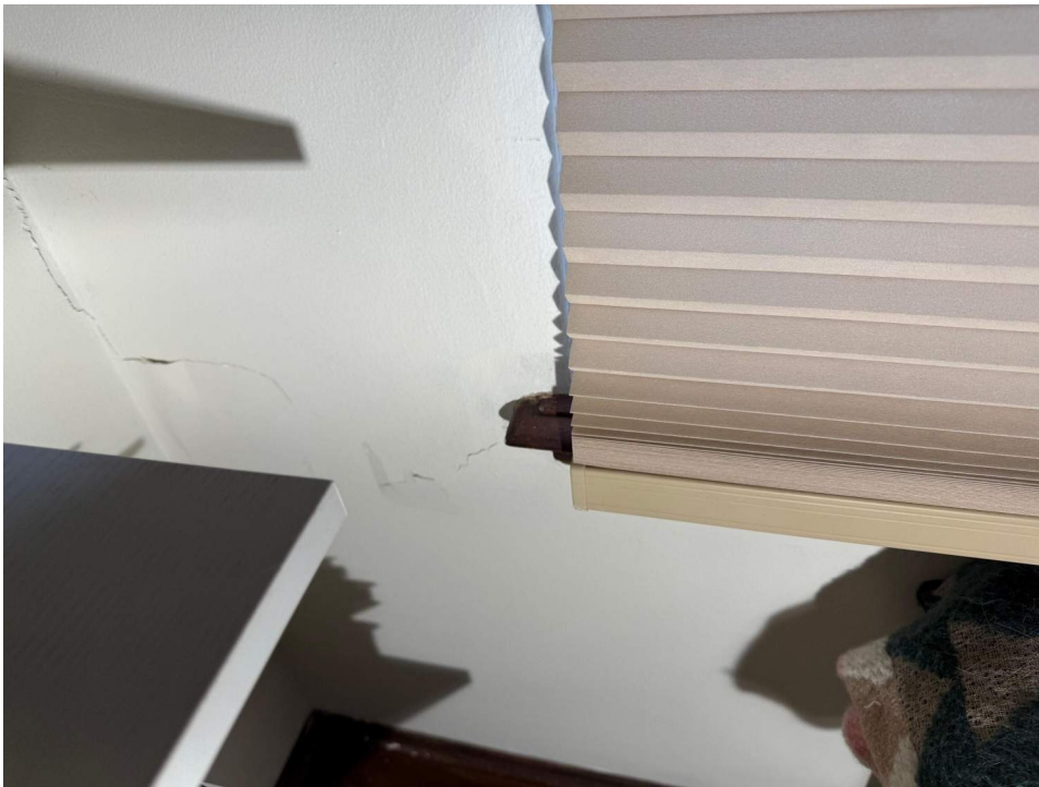
PHOTO 14: CRACKS IN EAST EXTERIOR WALL (UNIT 2)
