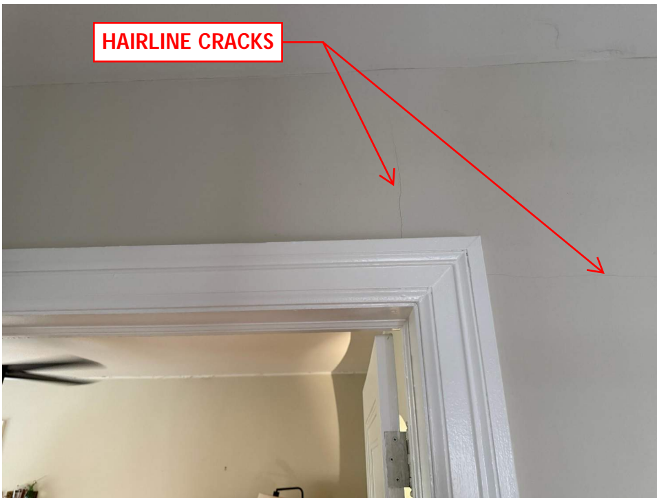
PHOTO 10: HAIRLINE CRACKS, TYPICAL (UNIT 4)
