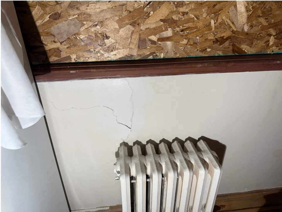
PHOTO 12: CRACKS IN NORTH EXTERIOR WALL (UNIT 2)
