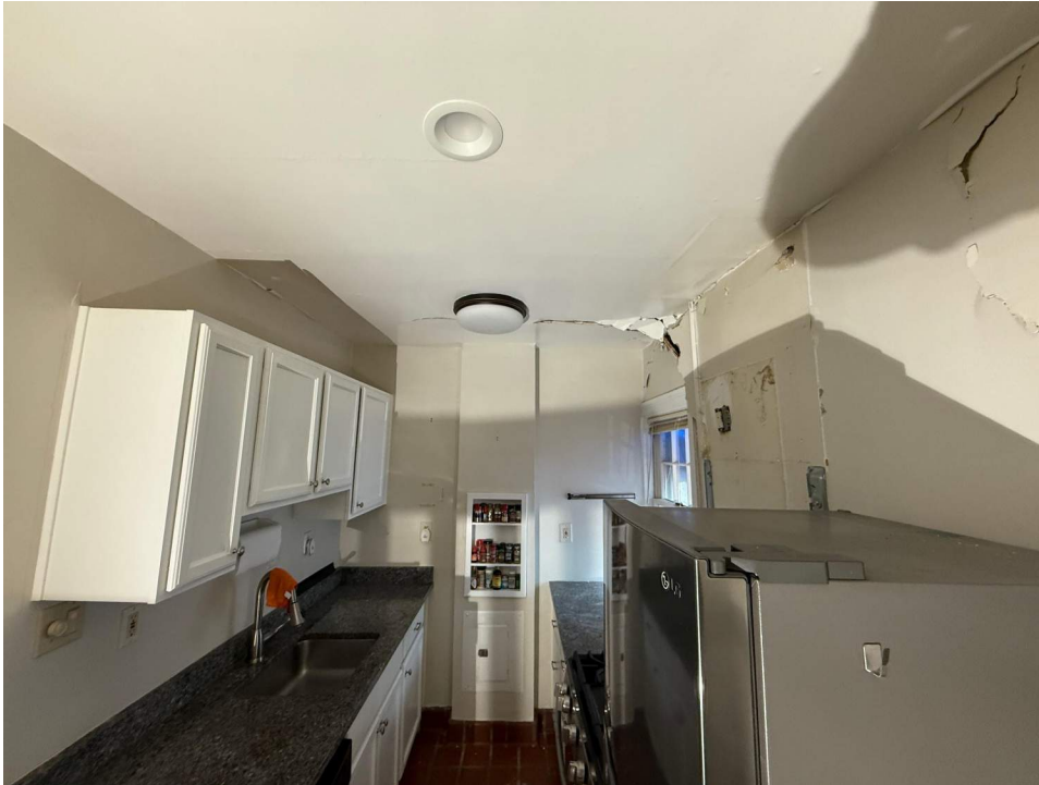
PHOTO 10: HAIRLINE CRACKS, TYPICAL (UNIT 4)
