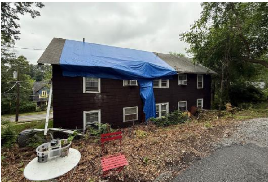
Figure 3: Rear elevation of the subject property showing the location of the chimney.
