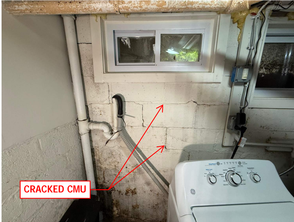
PHOTO 18: EXISTING CRACKS IN SOUTH CMU FOUNDATION WALL (BASEMENT)
