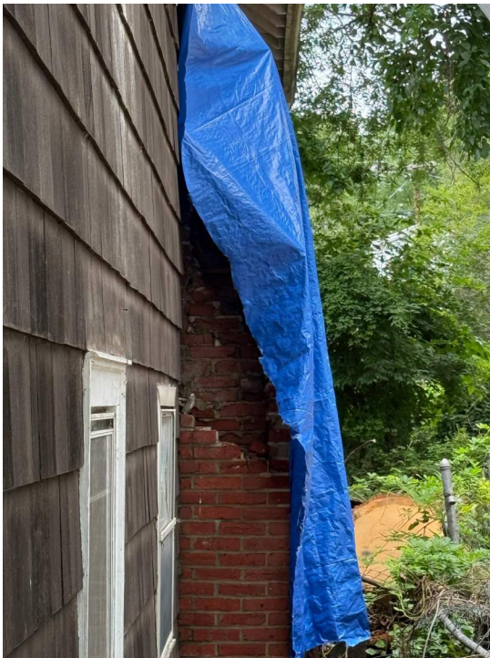
PHOTO 20: DAMAGED CHIMNEY
