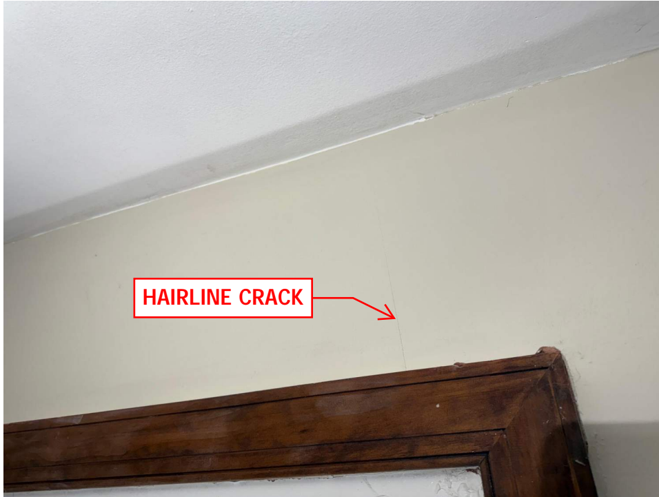
PHOTO 16: HAIRLINE CRACKS, TYPICAL (UNIT 1)
