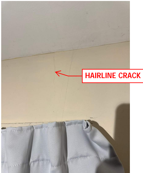
PHOTO 16: HAIRLINE CRACKS, TYPICAL (UNIT 1)
