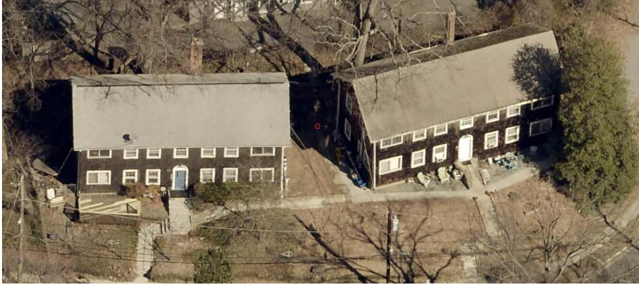
Figure 2: The subject property (left) and its twin showing the location and height of the chimneys.
