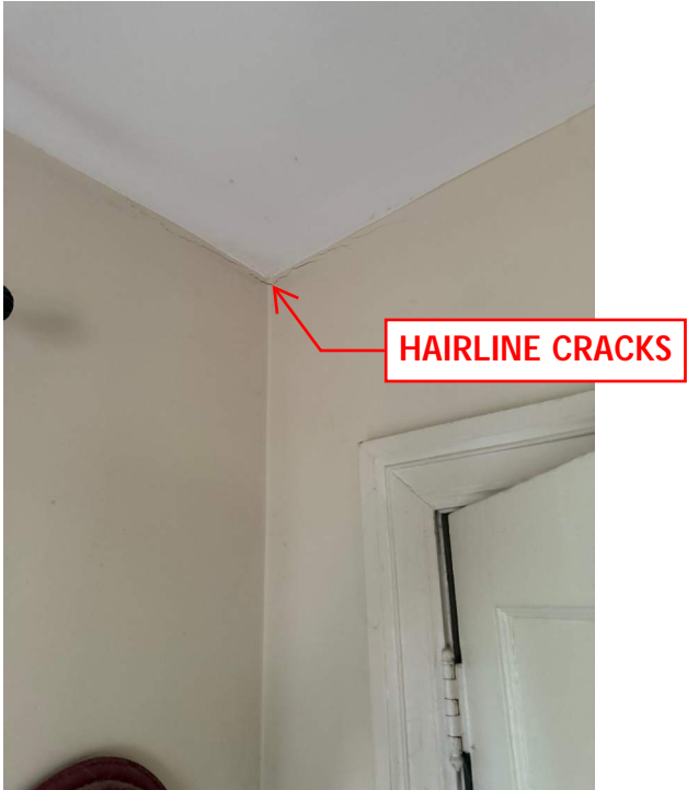
PHOTO 12: CRACKS IN NORTH EXTERIOR WALL (UNIT 2)
