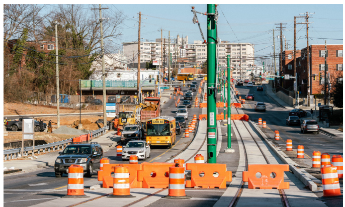
Purple Line Construction on Piney Branch Road
