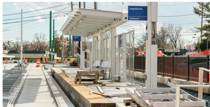
Purple Line Station Piney Branch Road Under Construction
