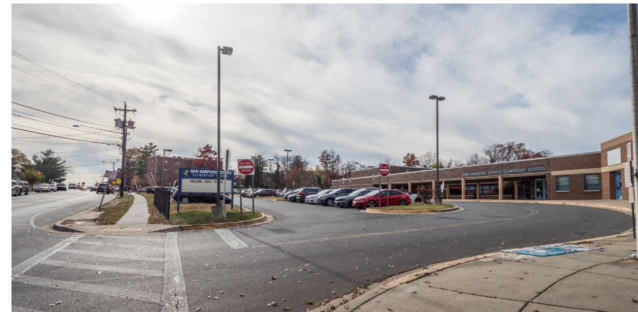
Schools in the Plan Area include Eastern Middle School (top) and New Hampshire Estates Elementary School (bottom)
