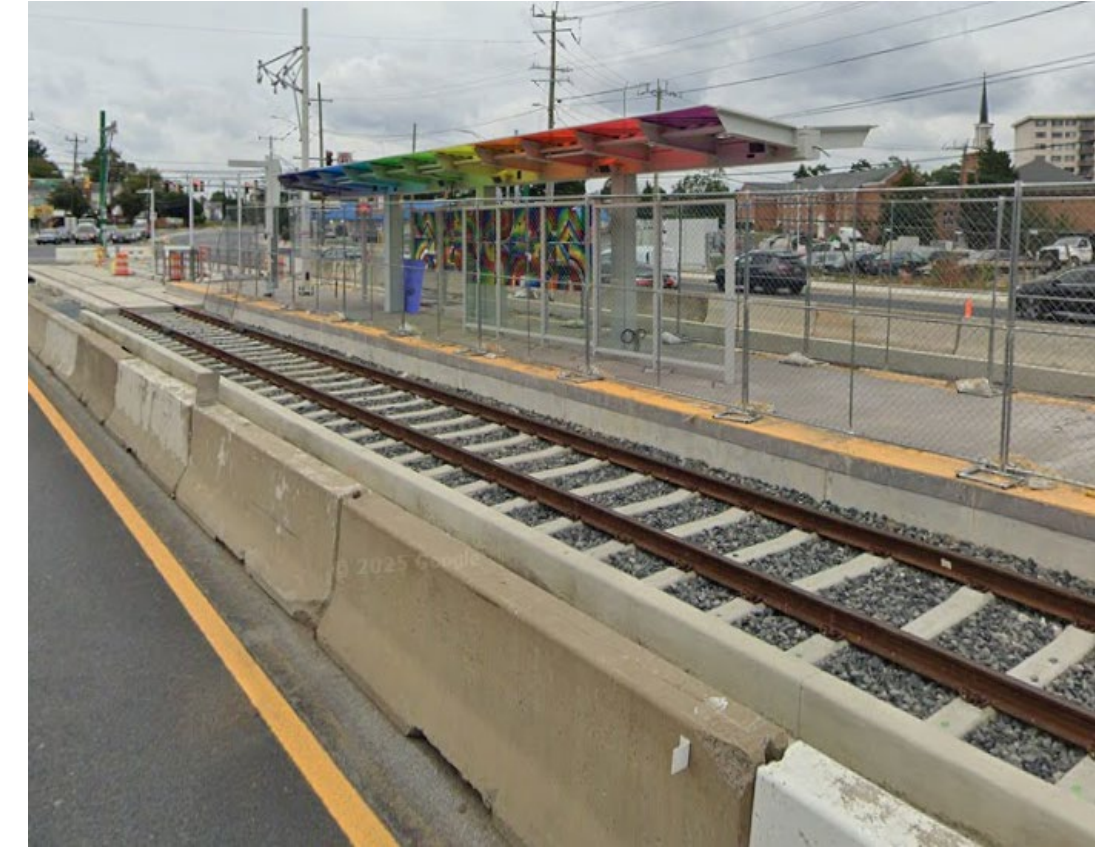
Piney Branch Road Purple Line Station (Under Construction)
