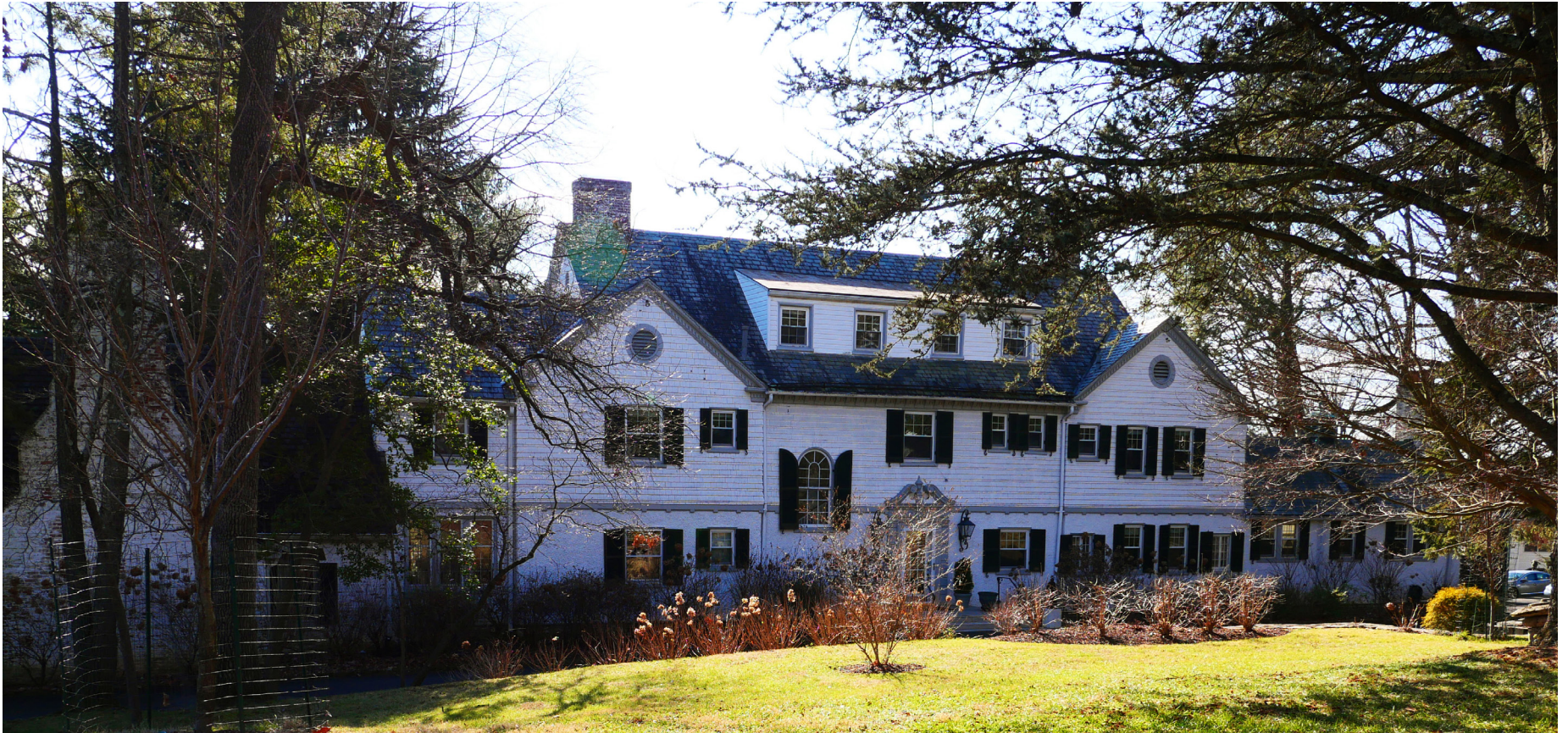
| Figure 1: View of Timberlawn from Sugarbush Lane, looking southwest (source: Montgomery Planning, 2023)
