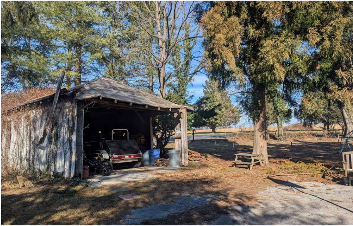
Figure 5: View of the southwest and southeast elevations of the existing garage. The location of the proposed garage is to the far right in the image.
