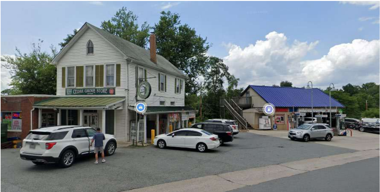
Figure 11: The Contributing Cedar Grove Store property at 23412 Ridge Road (left) and adjacent service station, which falls outside of the district boundary.
