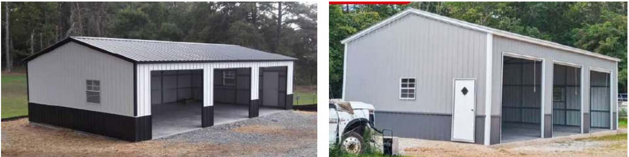
Figure 12: Examples of three-bay garages with 3/12 or greater pitched roofs, differentiated roofing, and corner boards.
