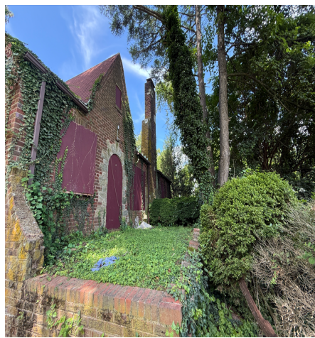
⑭ View of rear north facade at brick retaining wall
