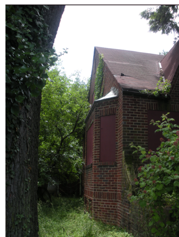
⑮ View of east facade with bay window visible
