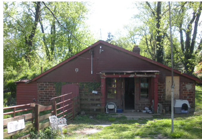
①⑥ Historic Kennel south facade facing Historic House
