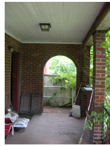
⑪ View at front porch looking east
