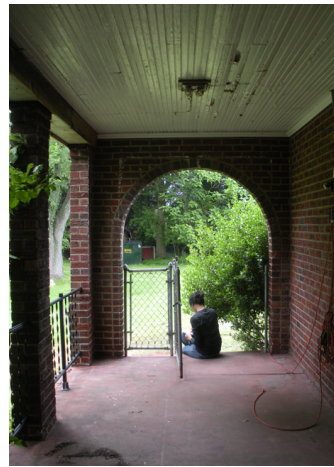
⑩ View at front porch looking west
