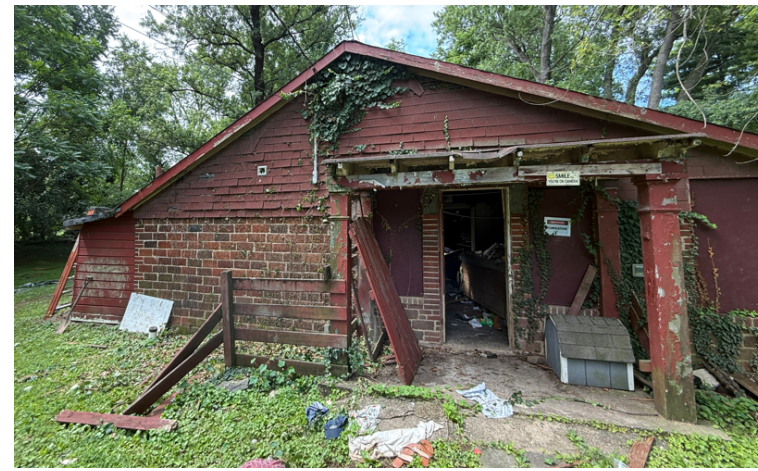
①⑦ Closeup of covered entrance
