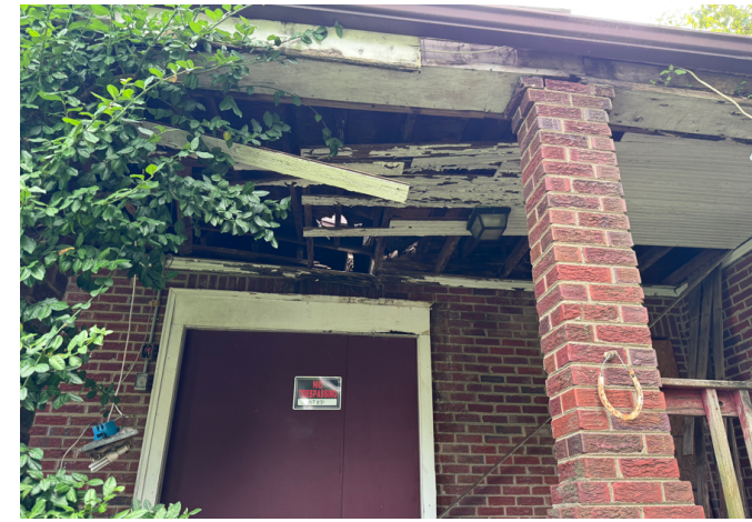
⑨ Closeup of current porch roof
