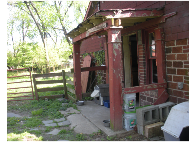
①⑧ Closeup of covered entrance
