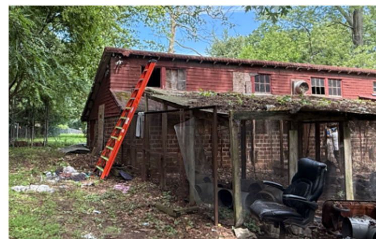
①⑬ View of east facade and angled view of north facade
