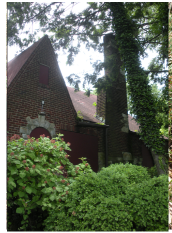
⑫ View of rear north facade
