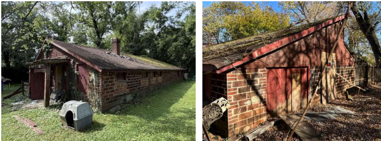
Figure 3: Views of the historic kennel building (from the applicant, left, and Historic Preservation Division, right).
