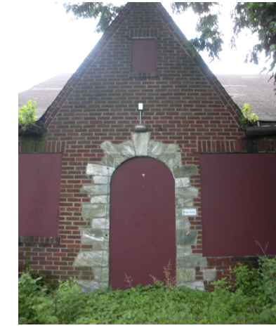
⑬ Closeup of rear door
