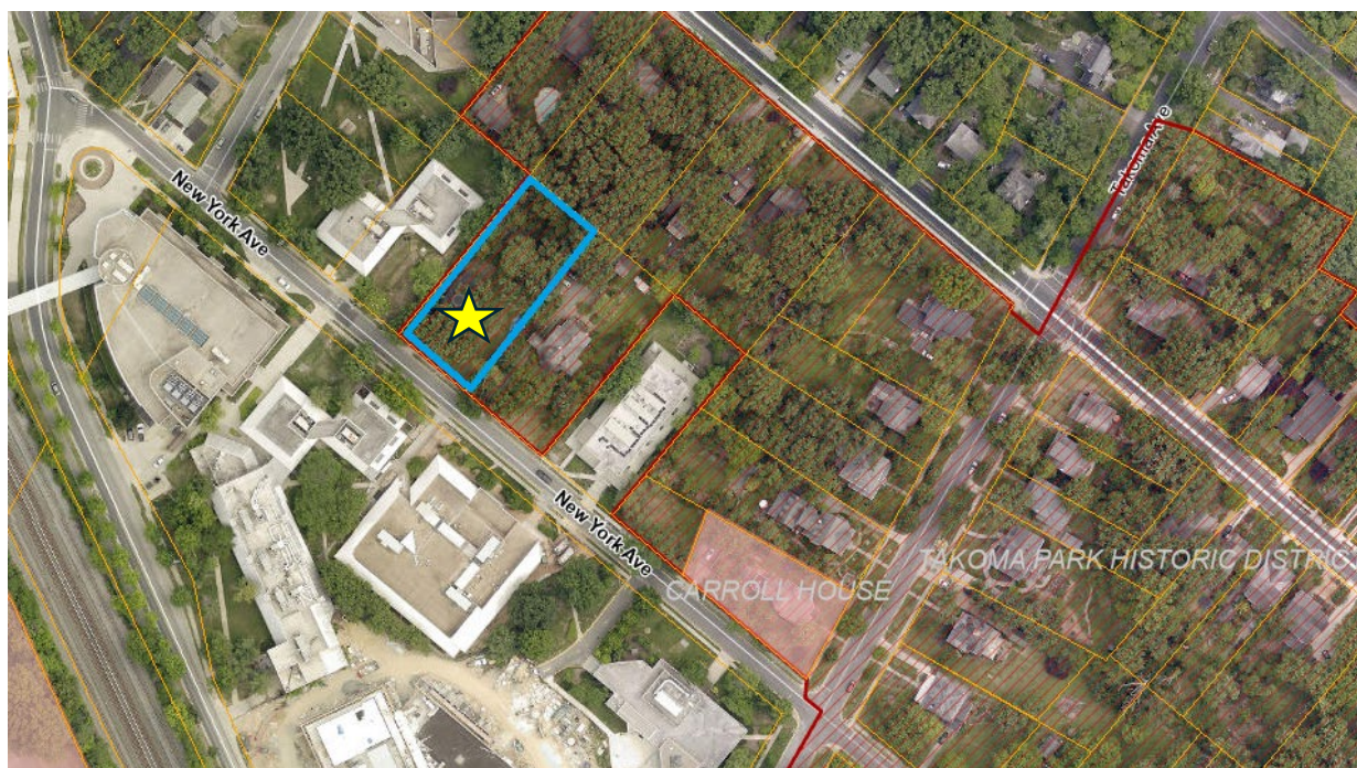
Figure 1: Location of the subject property (outlined in blue with a yellow star) within the Takoma Park Historic District (outlined and hatched in red).
