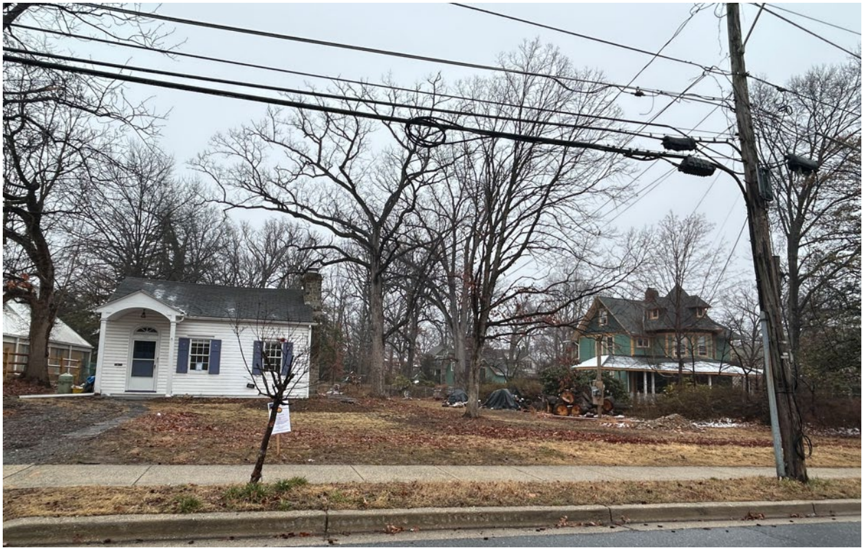
Figure 2: Front elevation of the existing Non-Contributing house at 707 New York Avenue, with the Outstanding resource on the adjacent parcel at 703 Takoma Avenue visible on the far right (March 2026, Historic Preservation Division).
