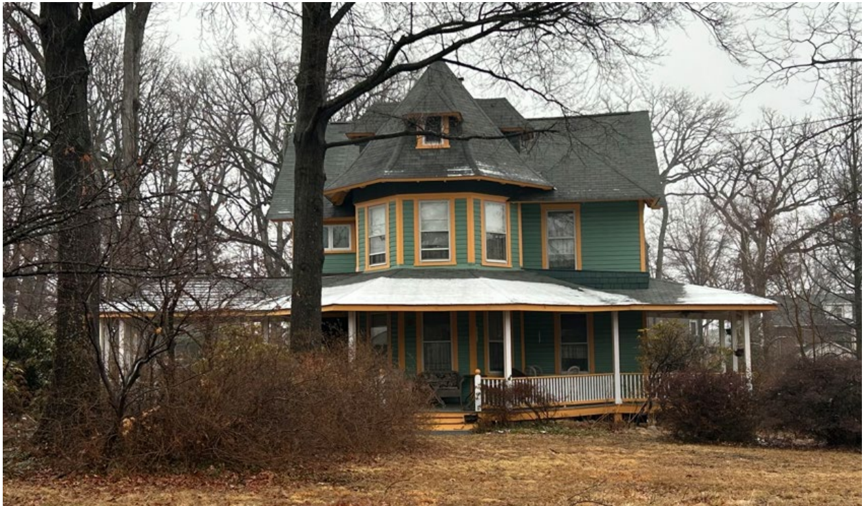
Figure 9: Front elevation of the neighboring Outstanding resource at 703 New York Avenue.
