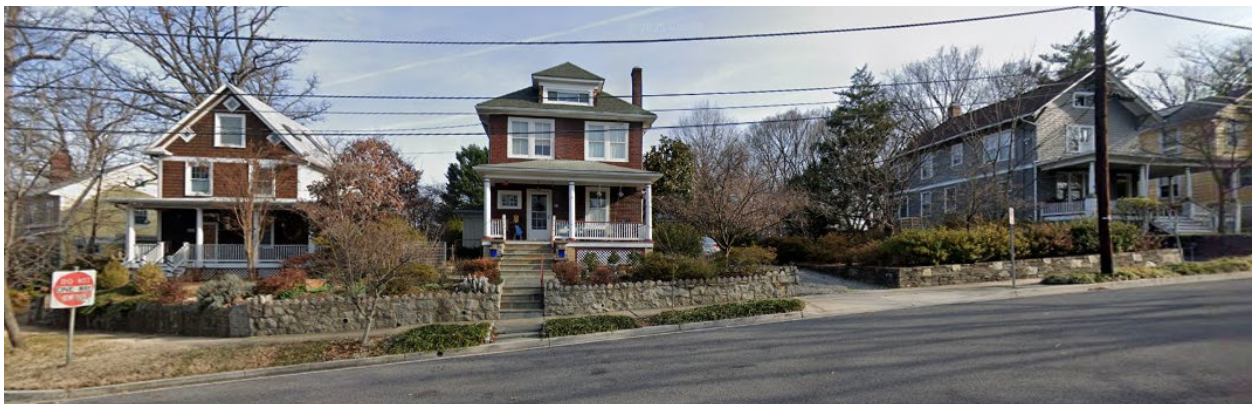
Figure 12: 239 Park Avenue, 16 Crescent Place, and 14 Crescent Place, showing additional roof forms found on 2.5-story houses in the district.
