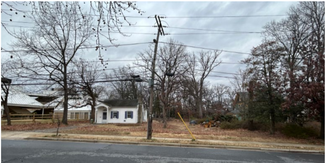
Figure 3: Front and partial side elevation of the existing Non-Contributing house at 707 New York Avenue, with the Outstanding resource on the adjacent parcel at 703 Takoma Avenue visible on the far right (December 2025, Historic Preservation Division).
