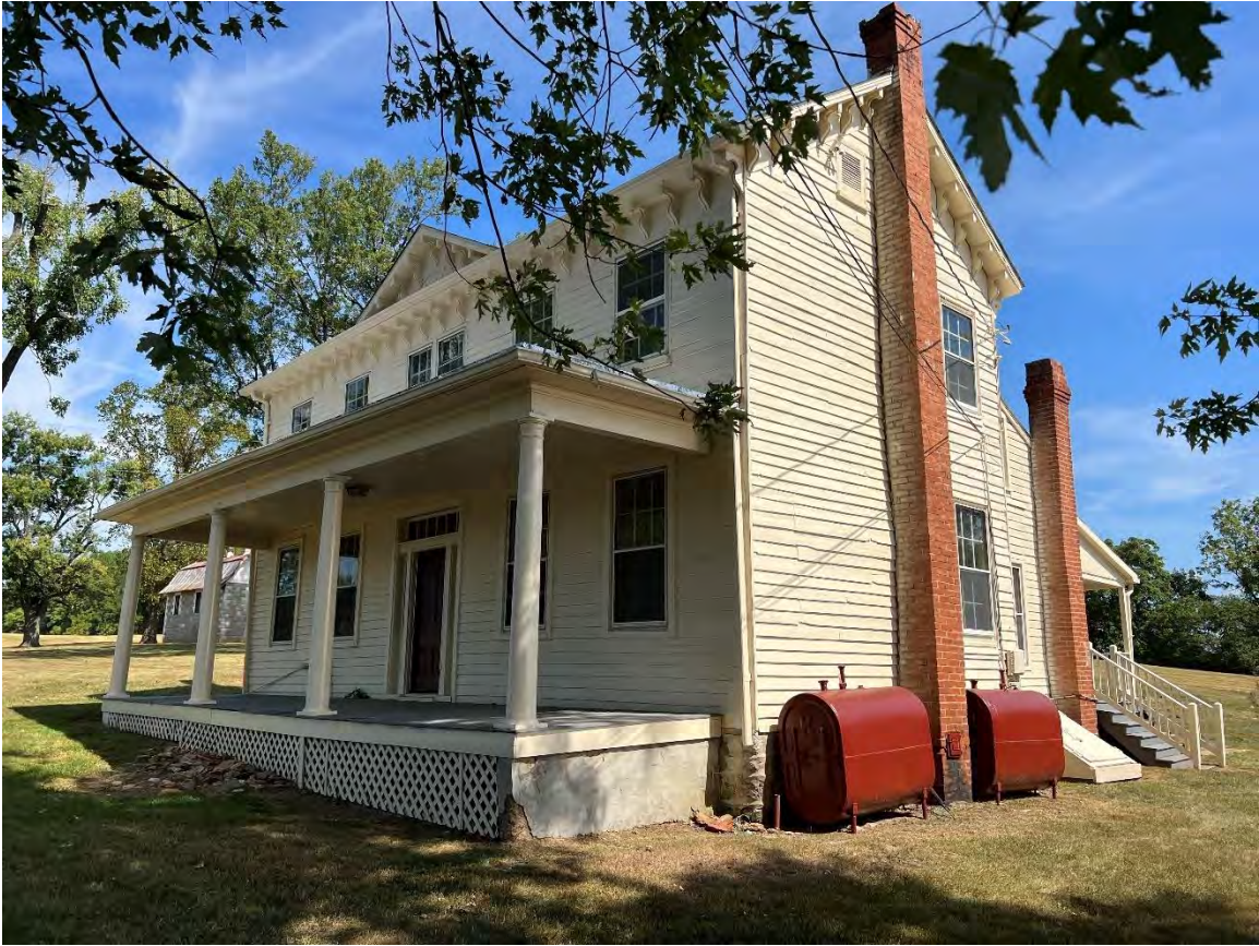
Photograph 1 – View of front and side building elevation.
