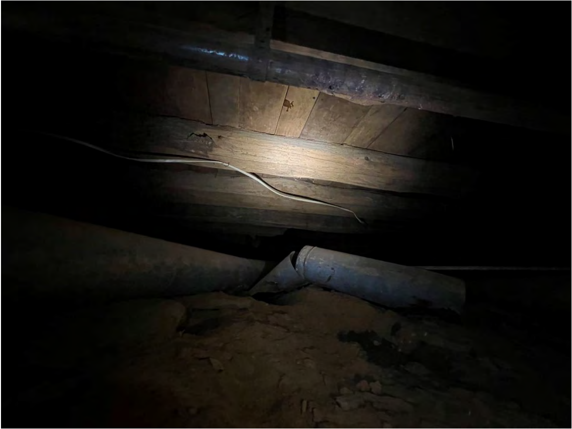
Photograph 7 – Typical log supporting first floor of Room 1C of addition.
