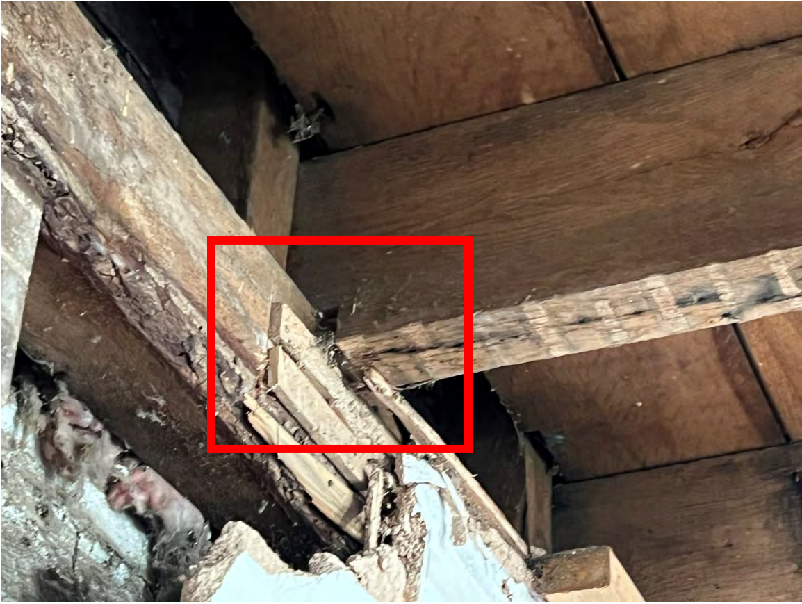
Photograph 19 – Typical notched floor joist.
