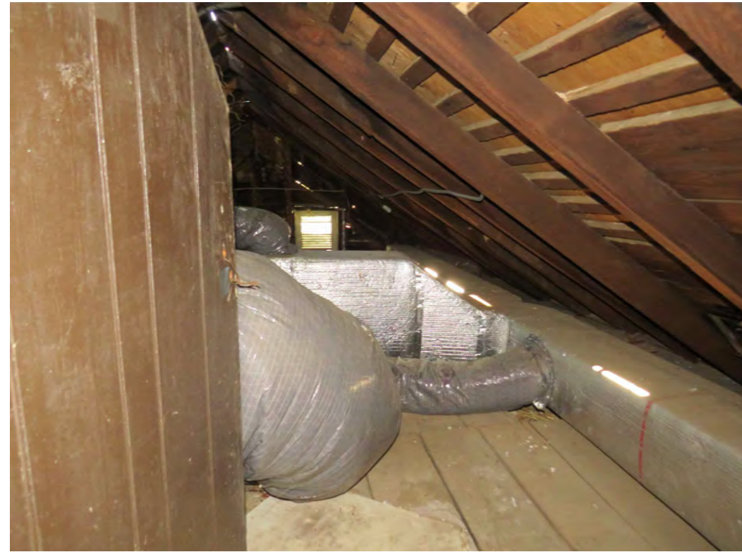
P3 ATTIC - W07 VIEW
