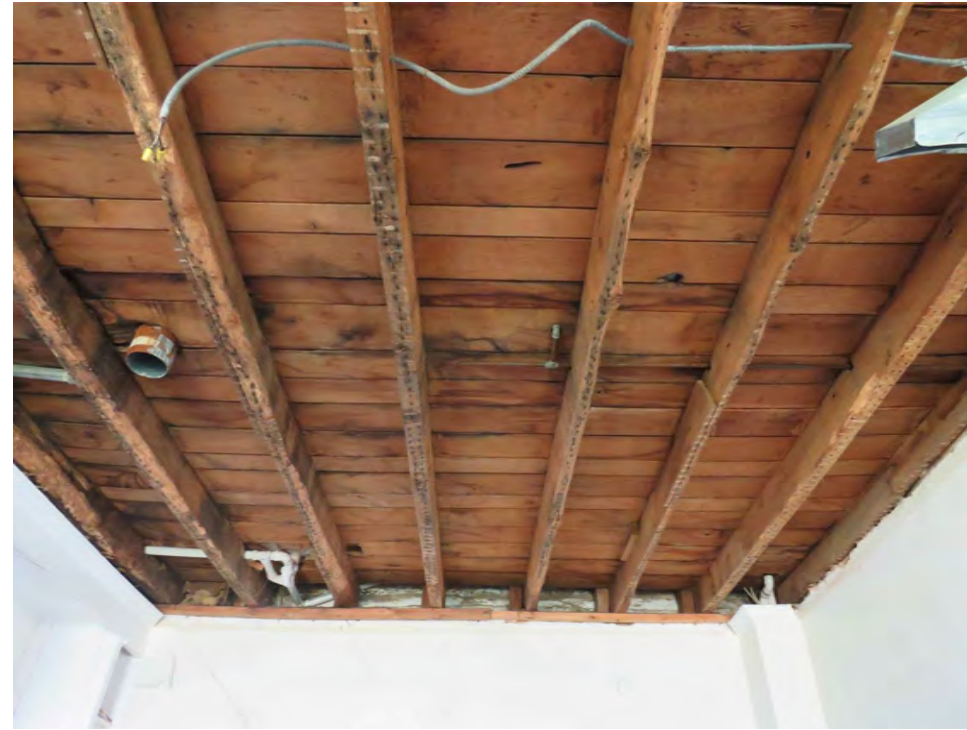
P ROOM 1A - CEILING
