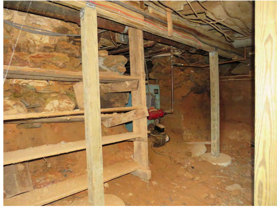
P BASEMENT - ROCK WALL VIEW 1
