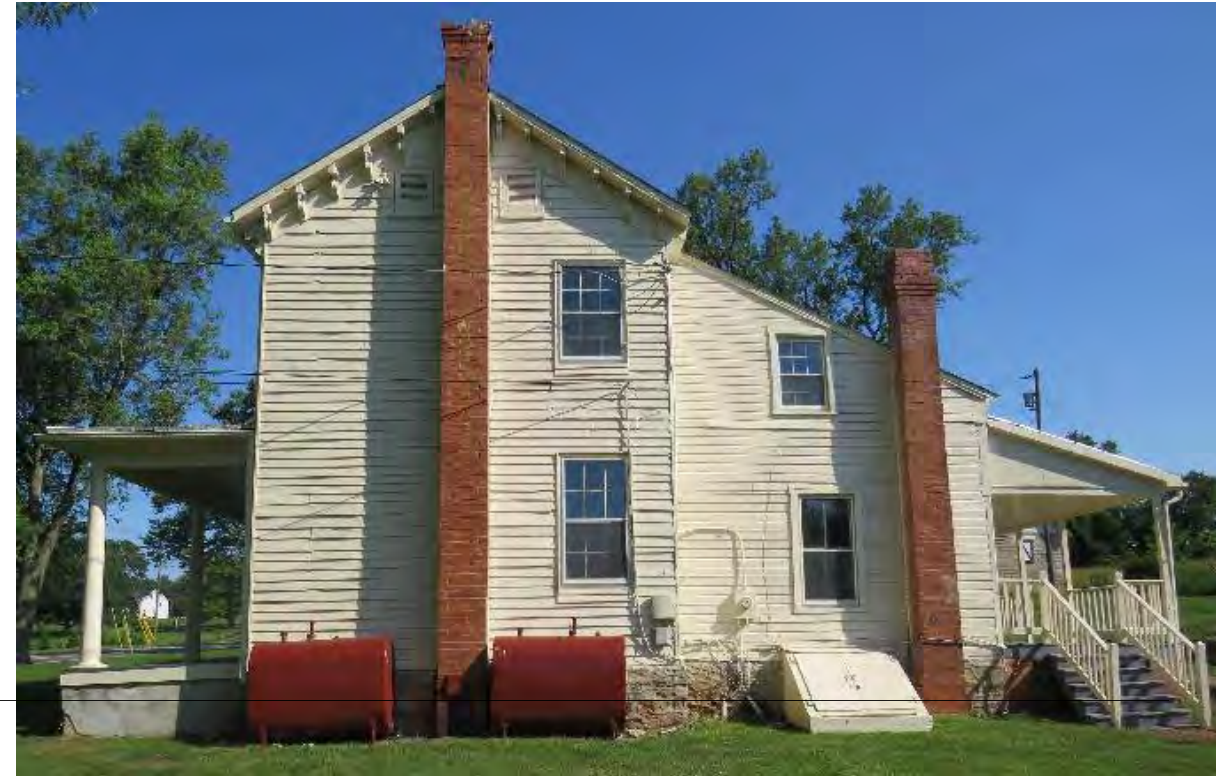
2. Right Side Elevation, 2025. Windows would be replaced in the front of the house. The rear portion of the house, including the back porch and the hatch access to basement, would be built new, with 6/6 windows and modern siding. The kitchen window sill in the rear will be raised slightly. The rear chimney would not be rebuilt.
