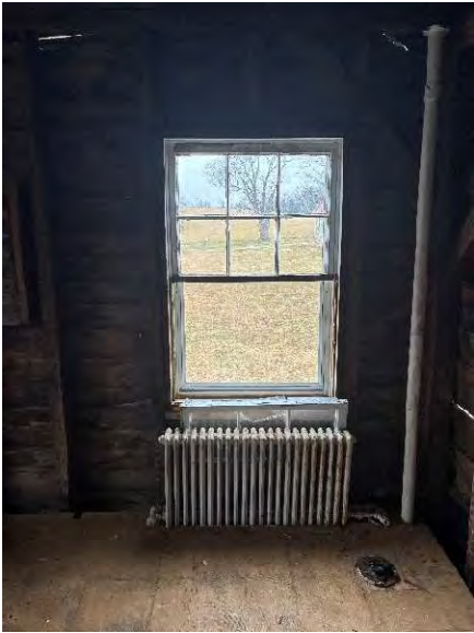
North Elevation 2nd Floor Window N2_2:
