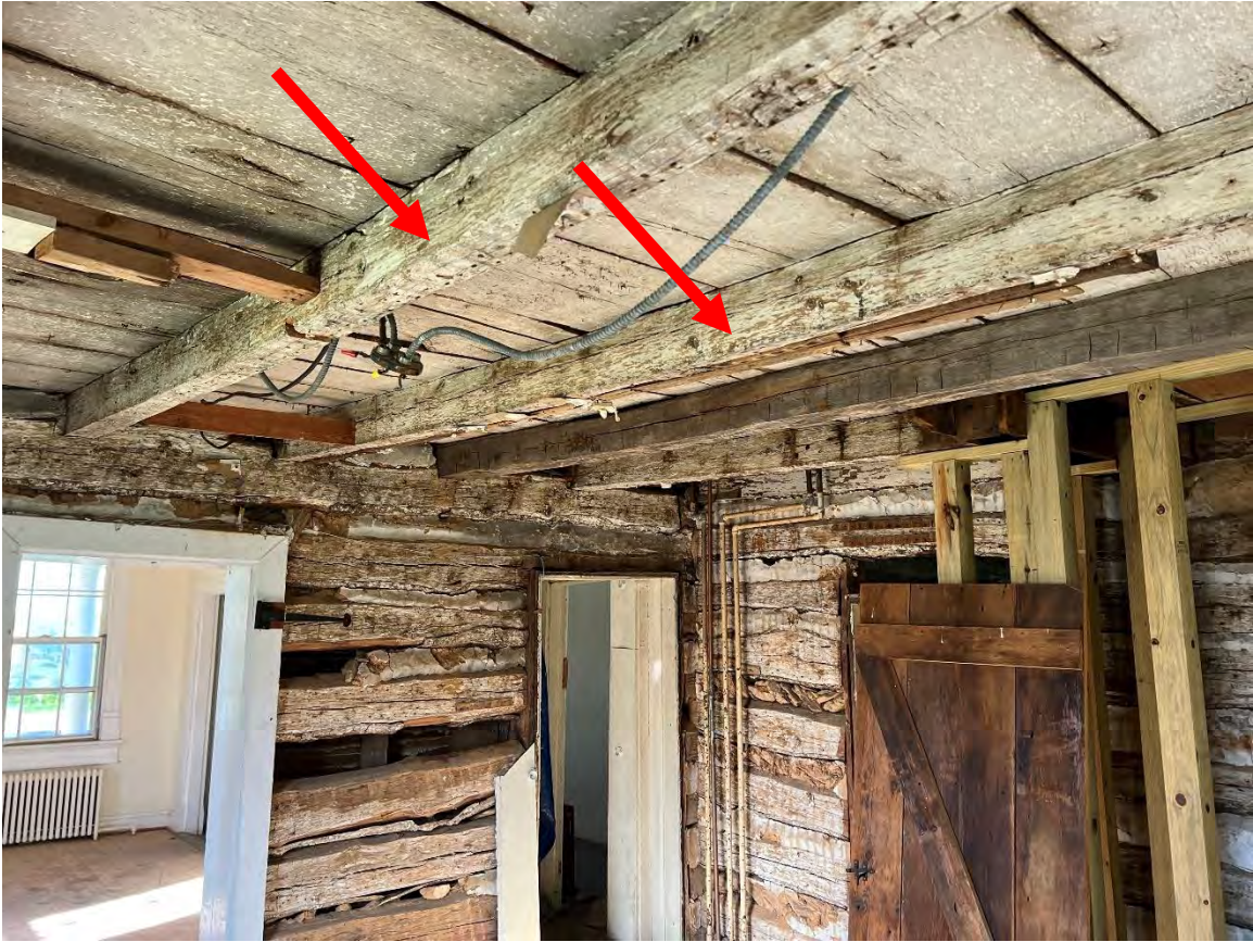
Photograph 15 – Typical timbers supporting 2 nd floor above log house.
