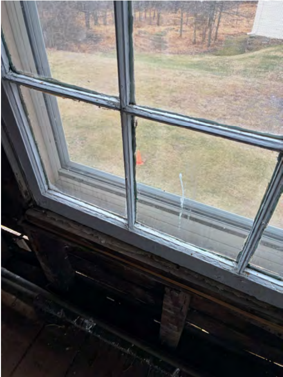
South Elevation 2nd Floor Window S2_1:
