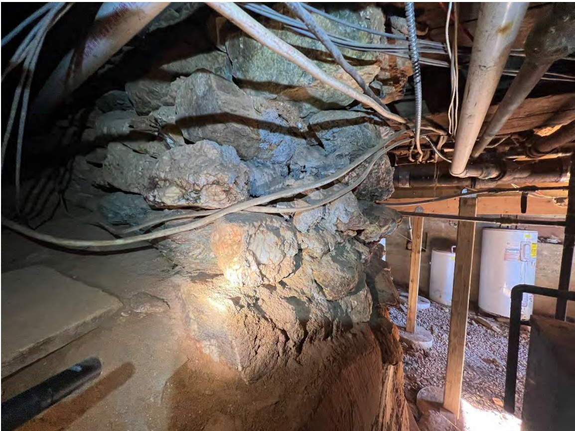
Photograph 6 – Typical stacked stone foundation wall.
