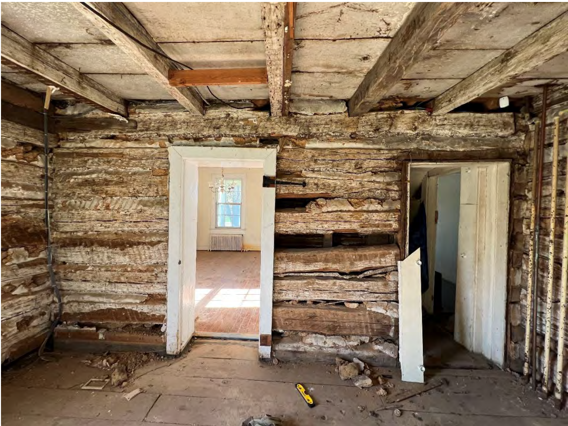
Photograph 12 – Typical rough openings are not square.
