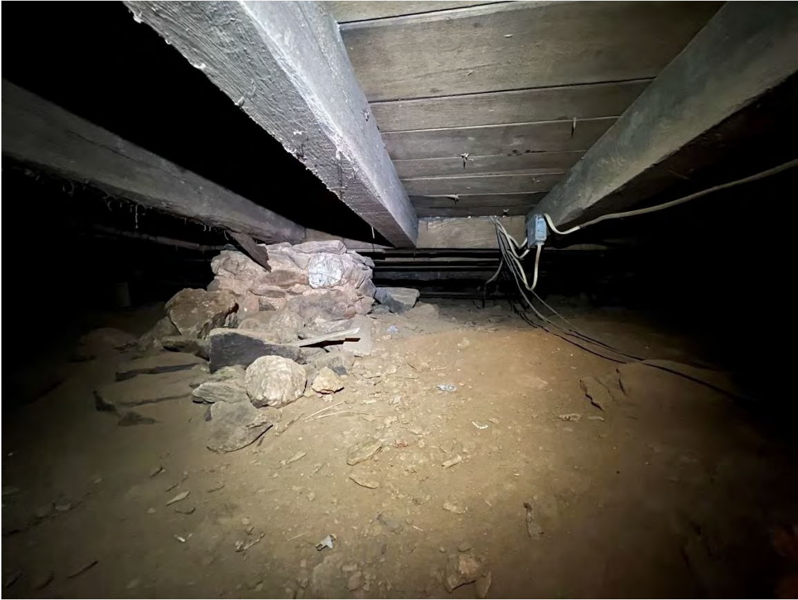
Photograph 9 – Typical deteriorated stone pier below addition.
