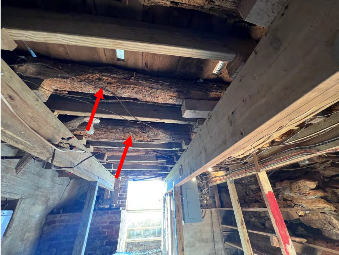
Photograph 3 – Typical original log house first floor framing (logs).
