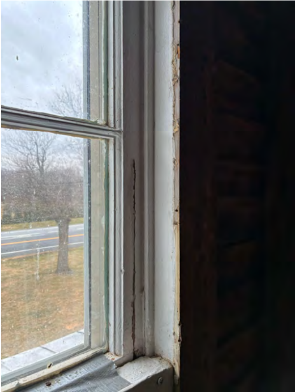
West Elevation 2nd Floor Window W2_2:
