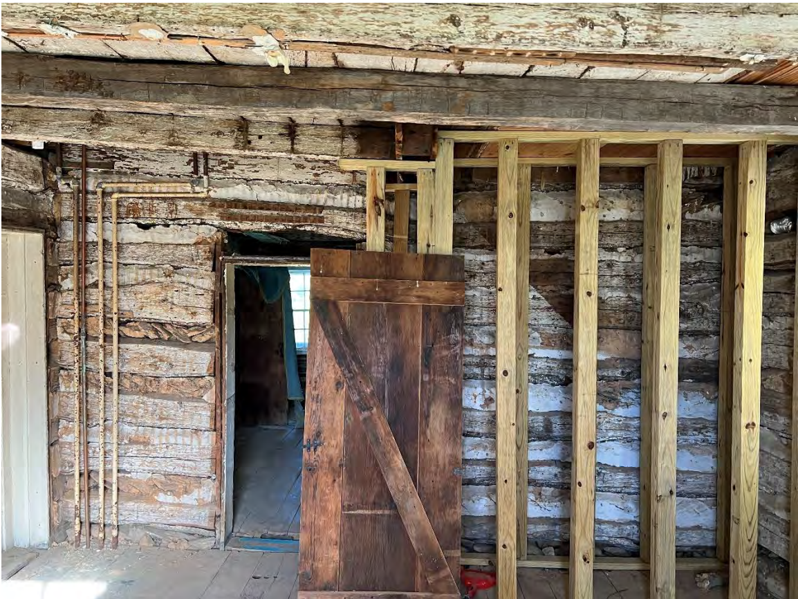
Photograph 16 – Temporary shoring installed in Room 1E.
