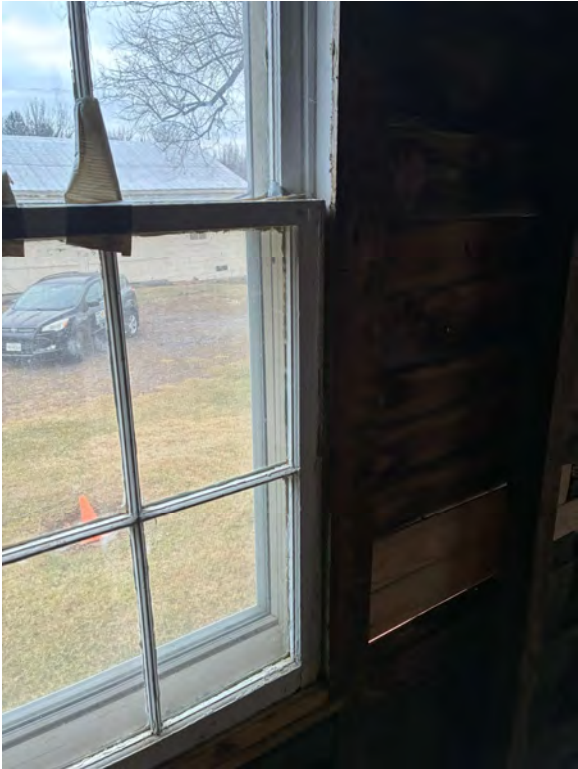
South Elevation First Floor Window S1_1:
