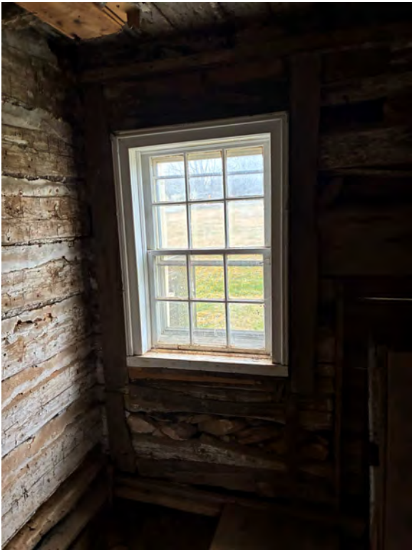
North Elevation First Floor Window N1_1:
