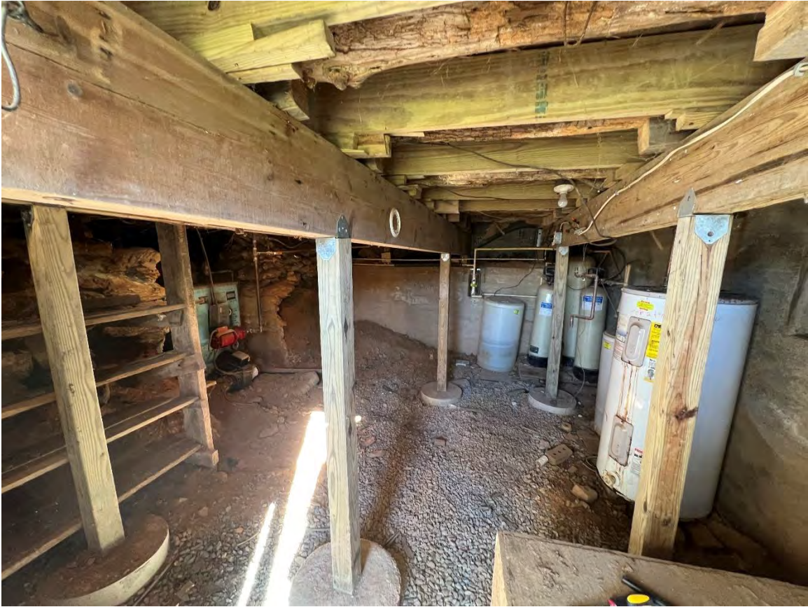
Photograph 5 – Typical supplemental framing beneath original log house.
