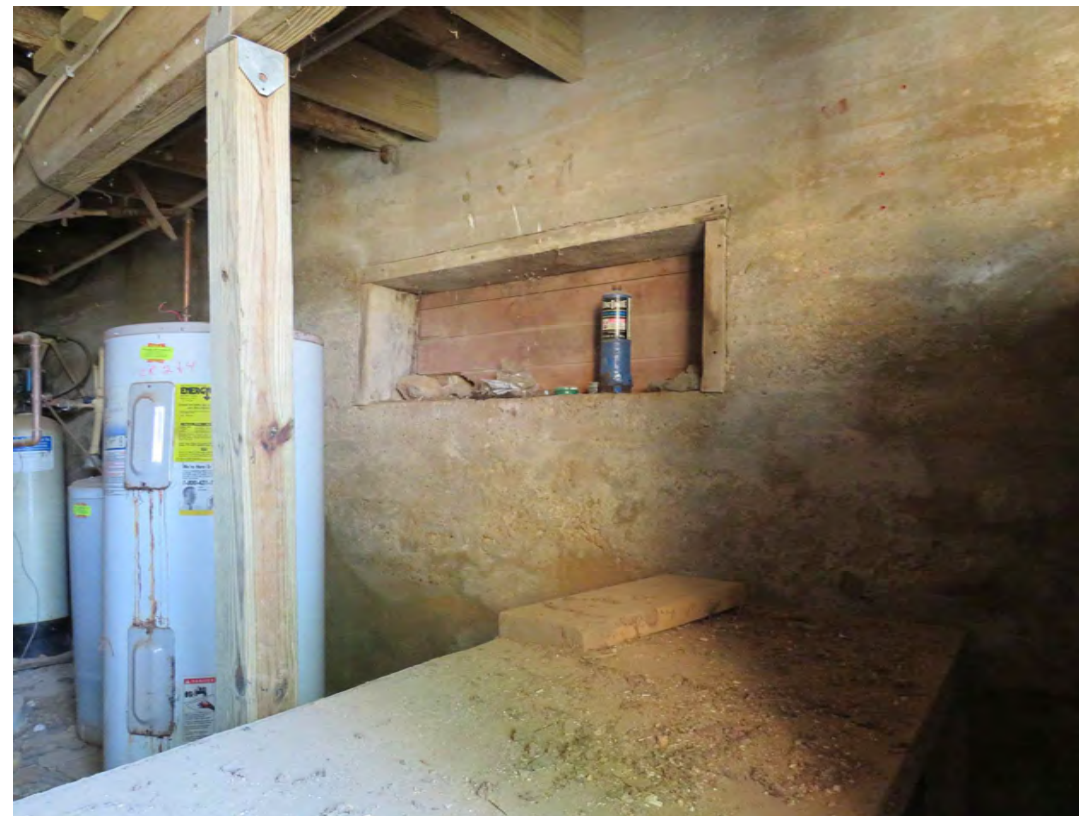
P BASEMENT - W10 VIEW
