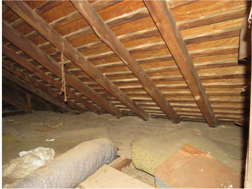
P ATTIC - W09 VIEW
