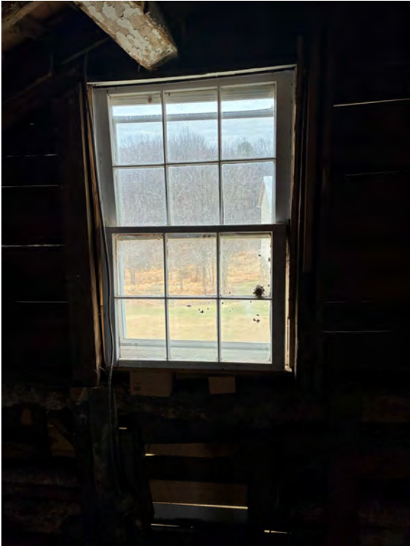
South Elevation 2nd Floor Window S2_2:
