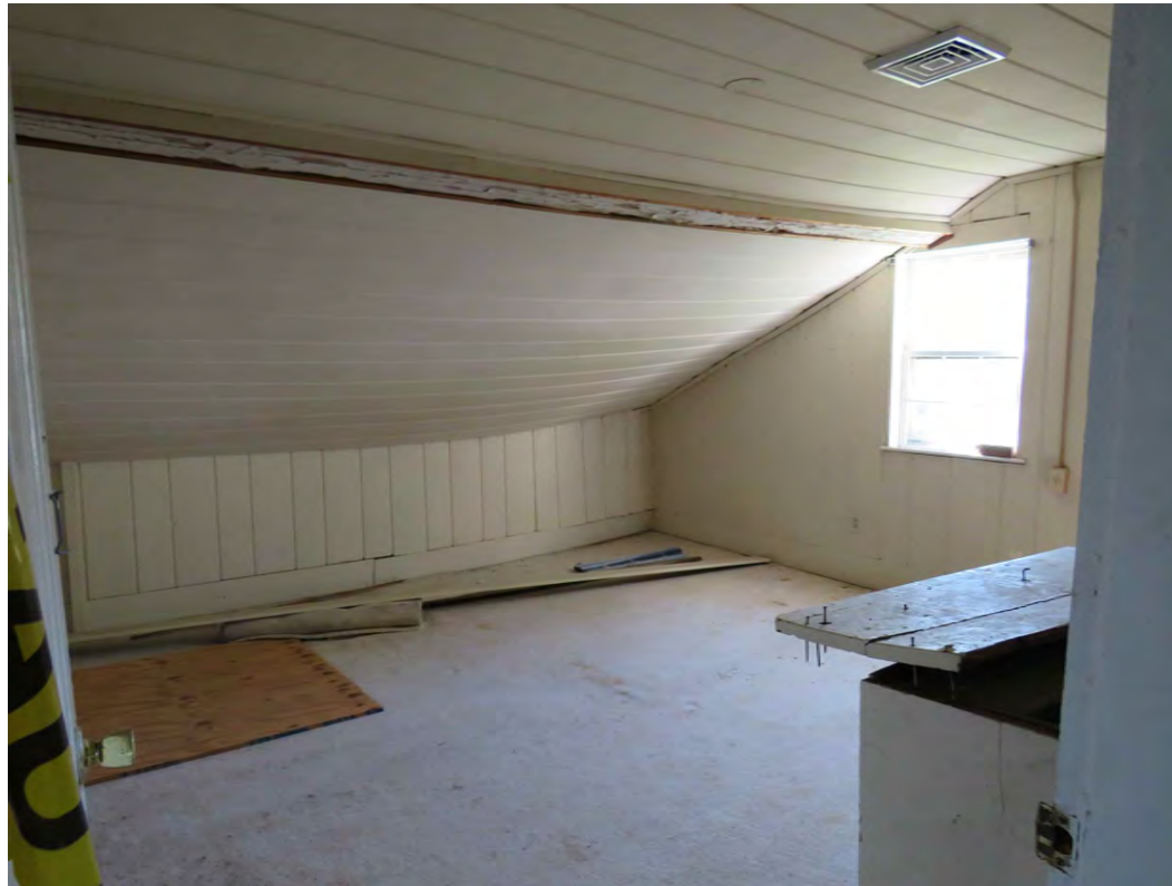
P 5 ROOM 2B - W11 VIEW
