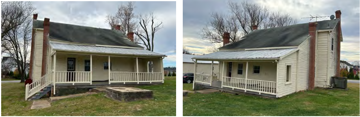
Figure 7: Existing rear elevation photographs.
