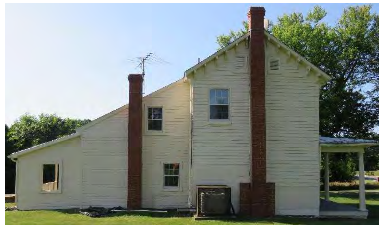
4. Left Side Elevation, 2025. Windows would be replaced in the front of the house and the siding repaired. The rear portion of the house, including the back porch, would be built new with 6/6 windows and modern siding. The rear chimney and the wing wall on the back porch would not be rebuilt.
