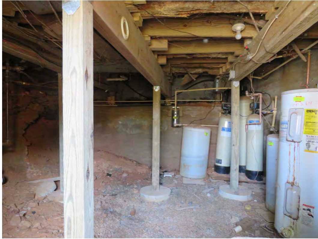
P 5 BASEMENT - EAST VIEW
