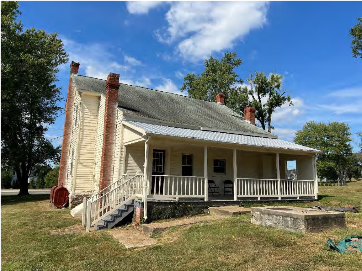
Photograph 2 – View of rear and side building elevation.
