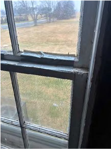
North Elevation 2nd Floor Window N2_1:
