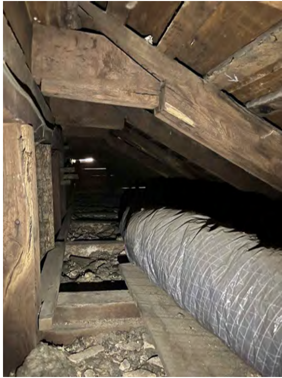
P3 LOG CABIN ATTIC - W07 VIEW
