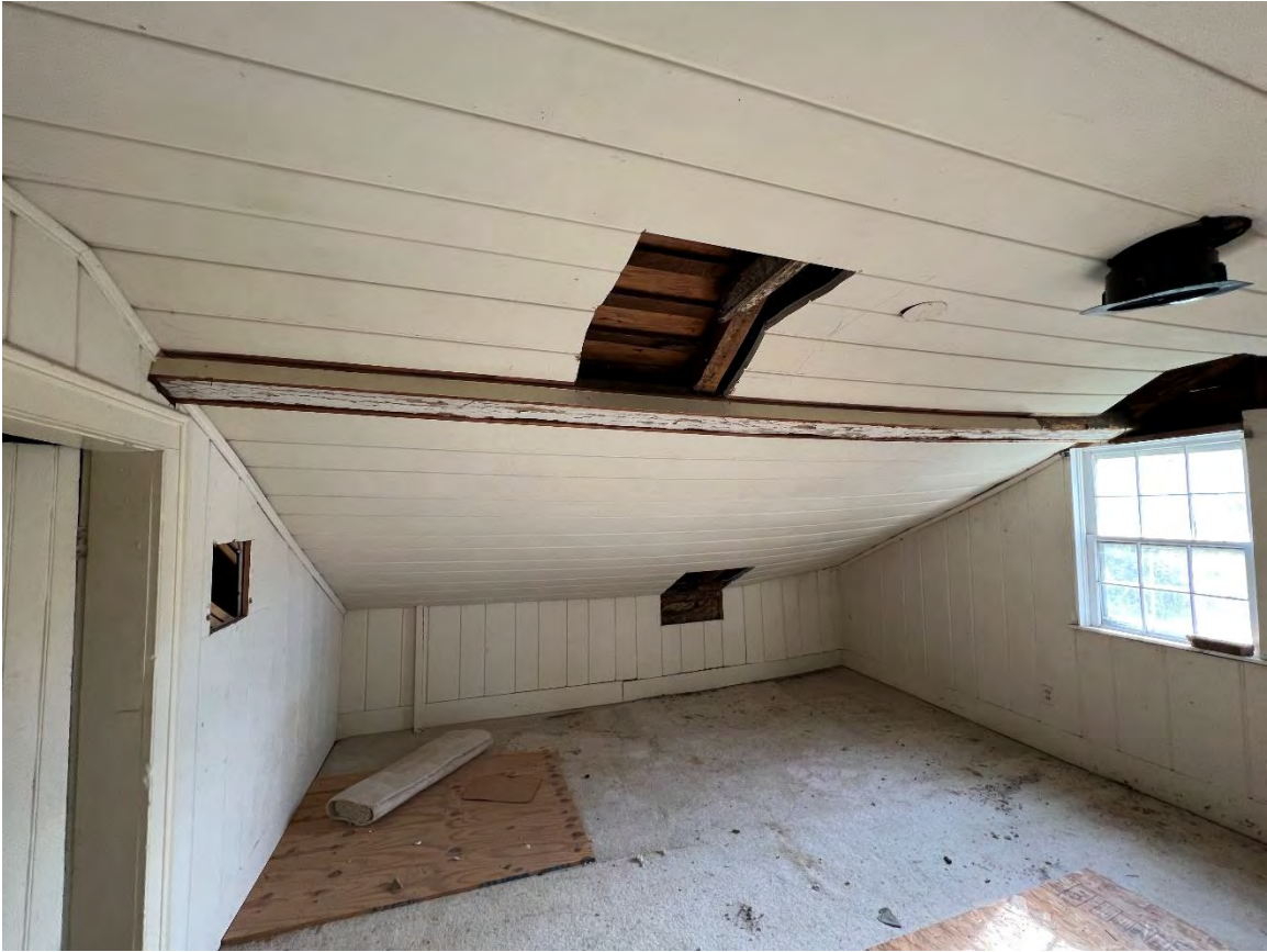
Photograph 21 – Intrusive sample locations in Room 2A.
