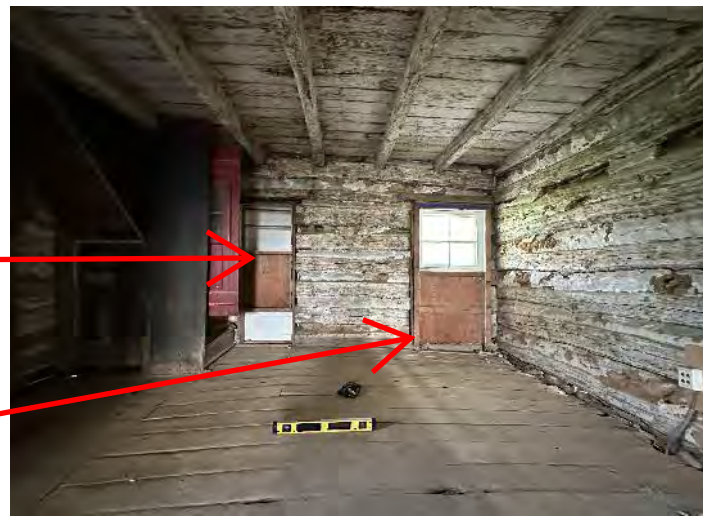
4. Interior view of previous door openings.
