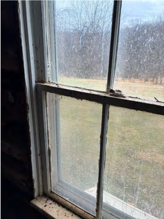
South Elevation First Floor Window S1_2:
