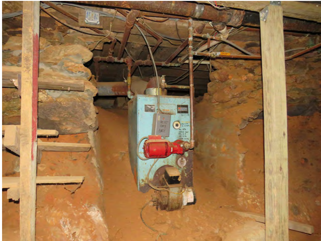
P BASEMENT - ROCK WALL VIEW 2
