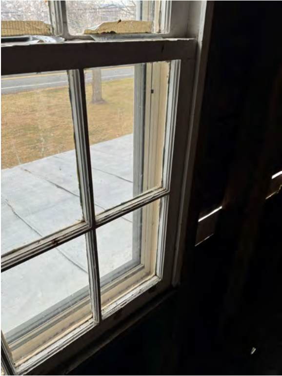
West Elevation 2nd Floor Windows W2_3 and W2_4:
