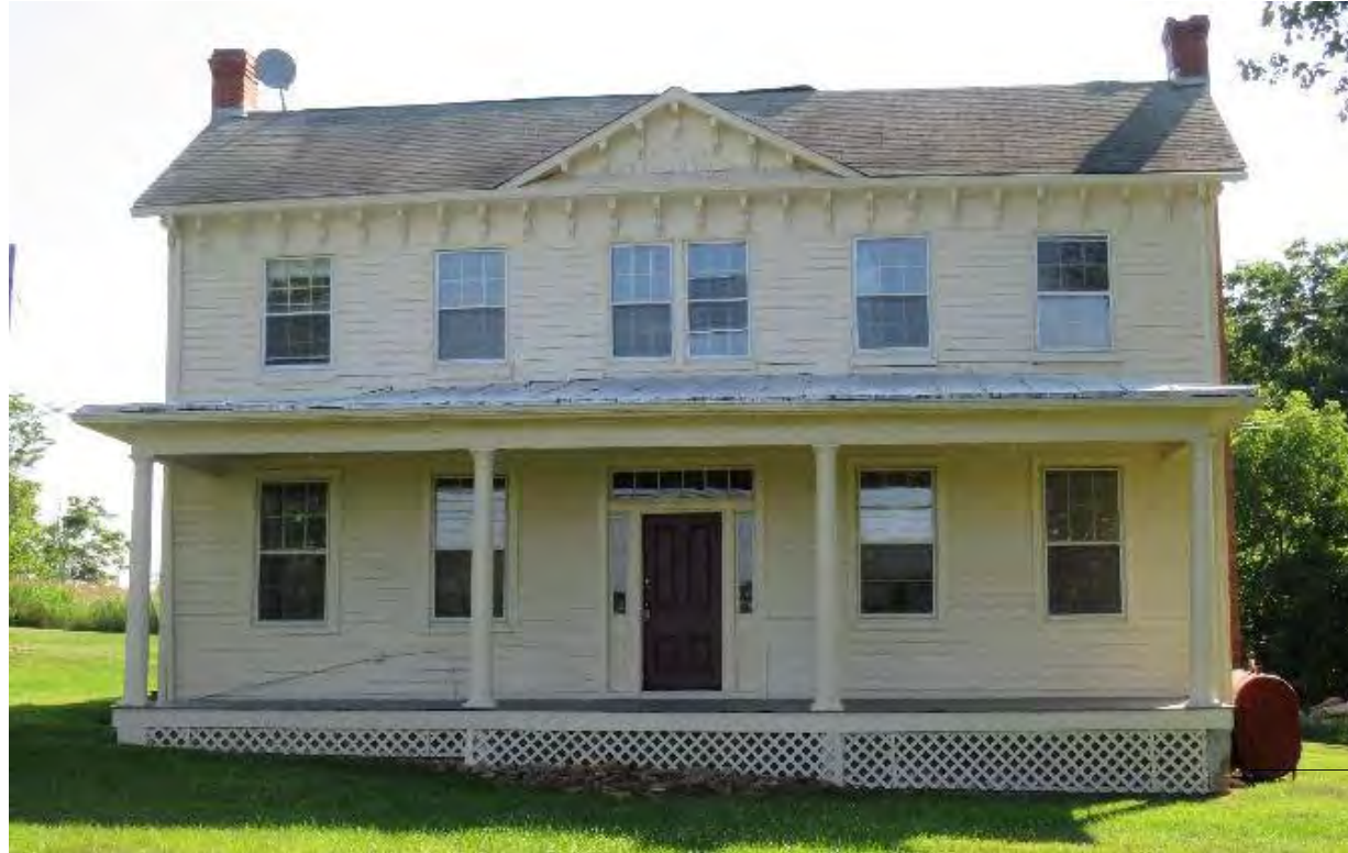
1. Front Elevation, 2025. Windows and roofing would be replaced and stairs would be added off the front porch.
