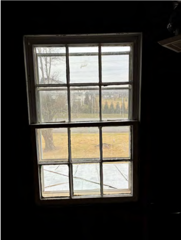
West Elevation 2nd Floor Windows W2_6
