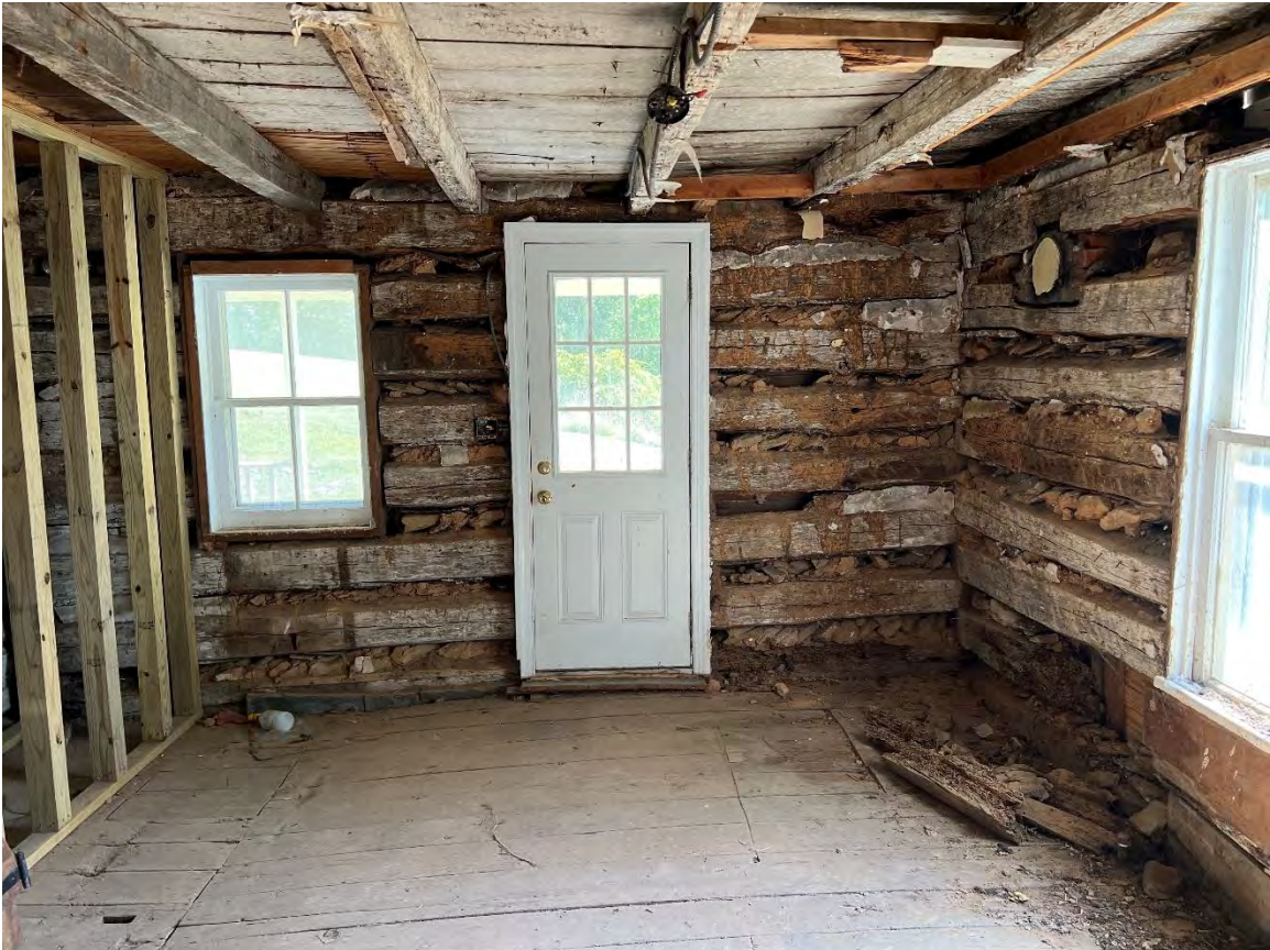
Photograph 10 – Typical view of log walls within log house interior.
